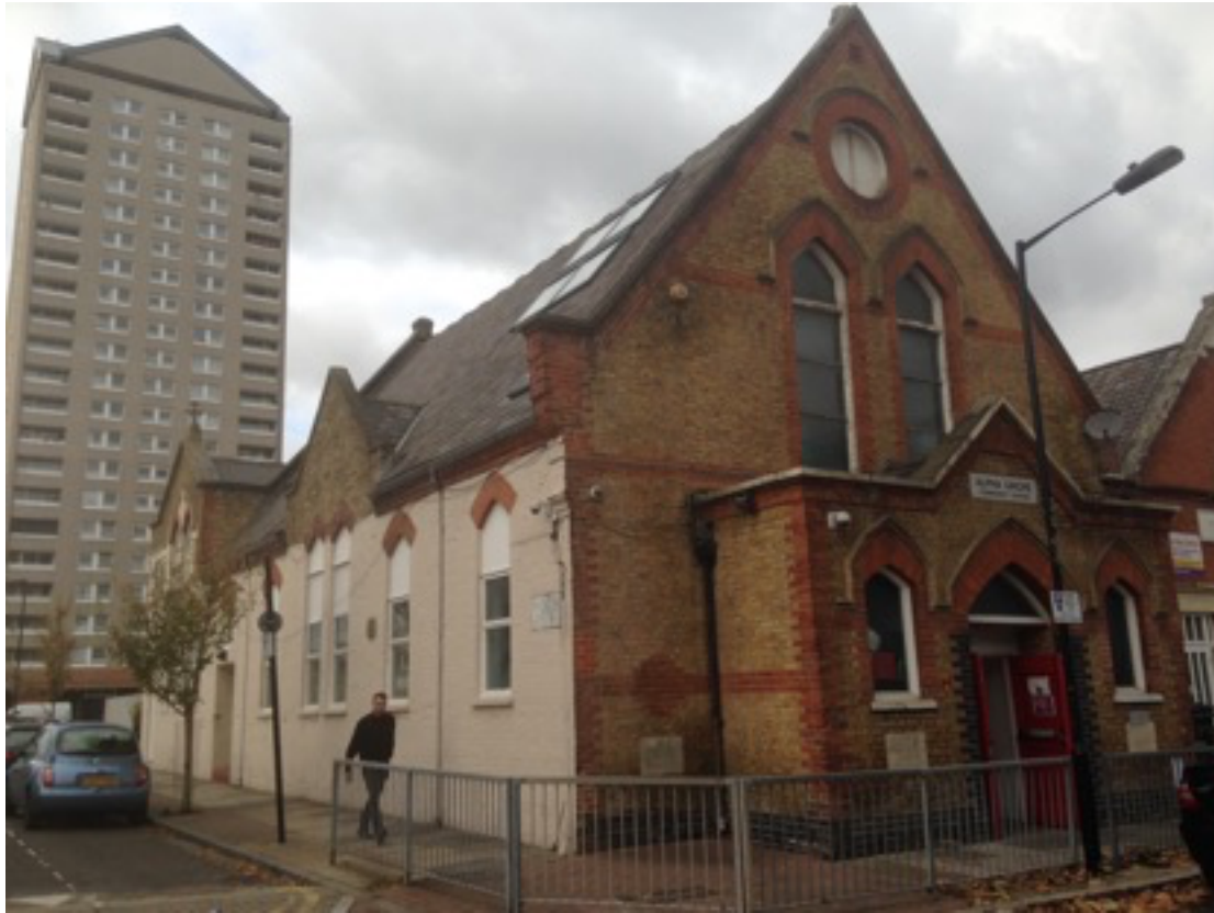
Figure 3: Millwall Chapel, Alpha Road. Built 1887, building now used as a community centre. Photograph by author 2016.
