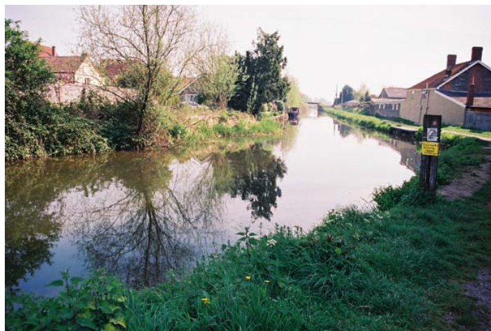
Plate 2.12: Bridgewater-Taunton Canal at Creech St. Michael (Picture by author).
