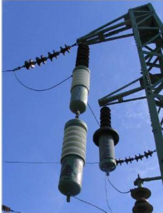
Fig 2.1 Coupling capacitors in the HV distribution network [figure abstracted from Kosonen, 2008].
