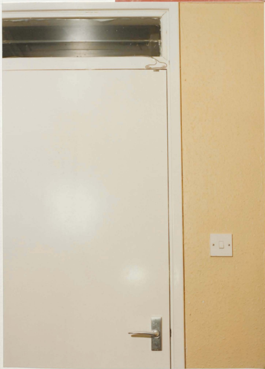
2:9 Magnetic switch on door lintel
