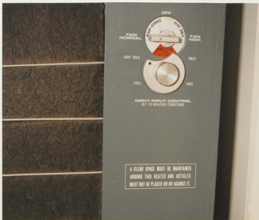
2:3 The charge control on the Electricaire
