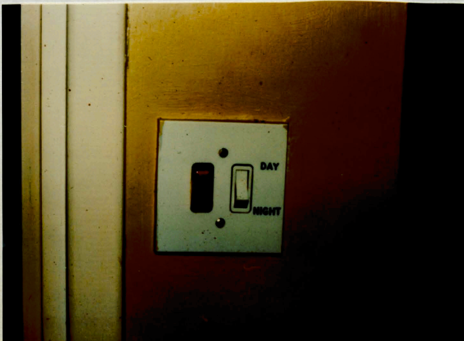
4:14 Mrs D's Day/Night control glowing red while the immersion- switch was "off"
