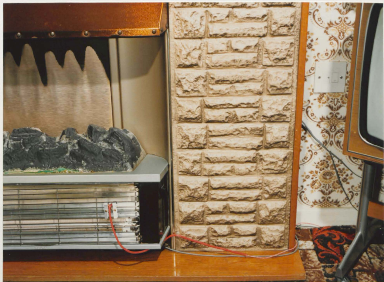
2:11 Electric fire fitted with heat- and light-sensitive switches
