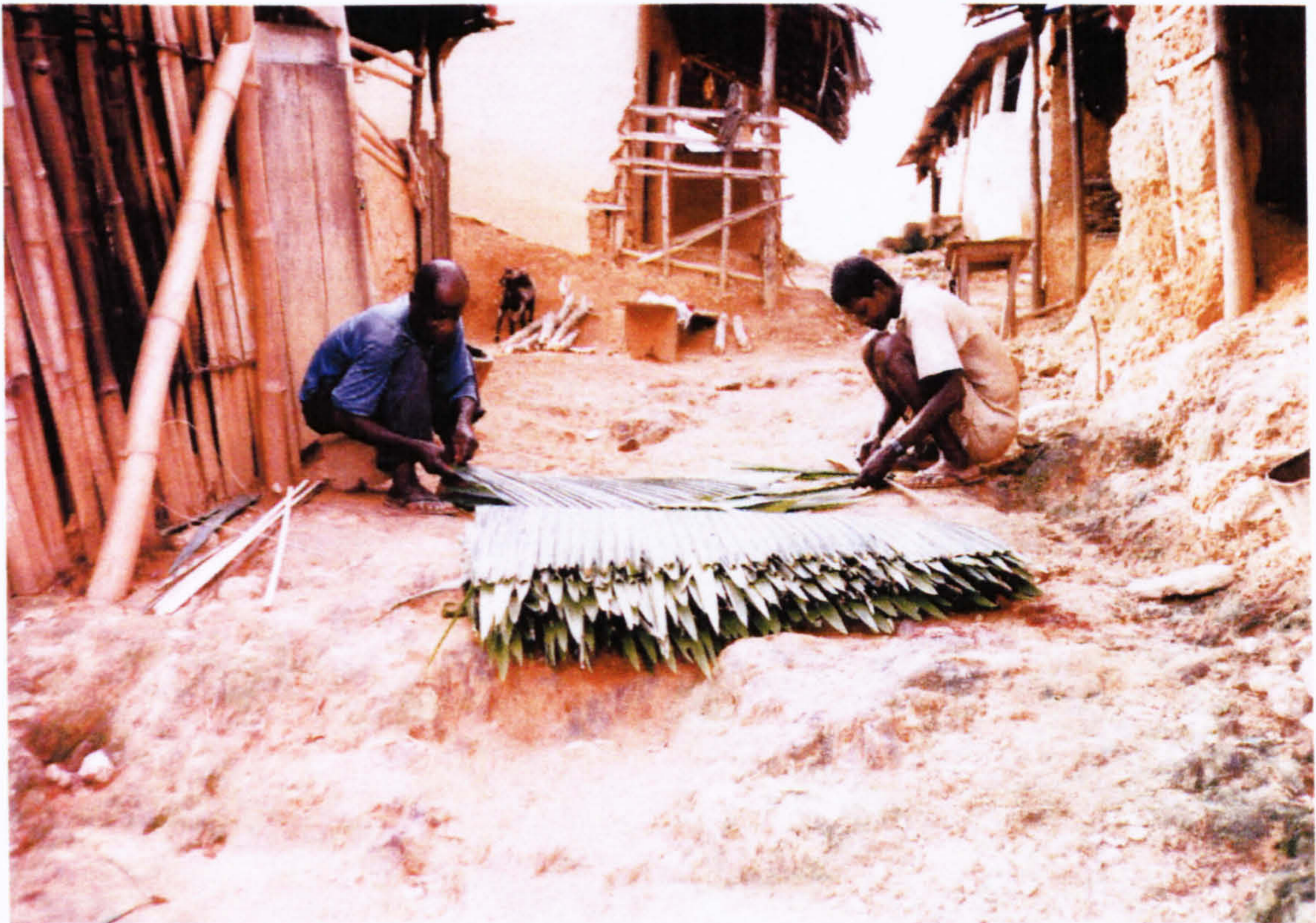
Plate 7.6. The use of raphia palm leaves for making roofing tiles (raphia thatch).
