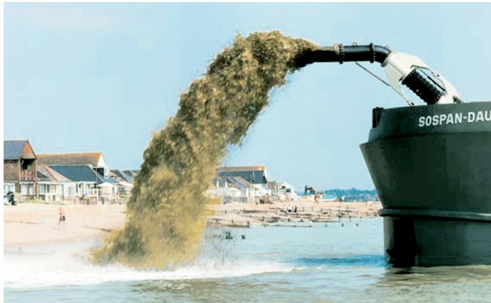
Figure F7 An offshore rainbow dredger replenishing Pevensey Bay in East Sussex (Website 22)
