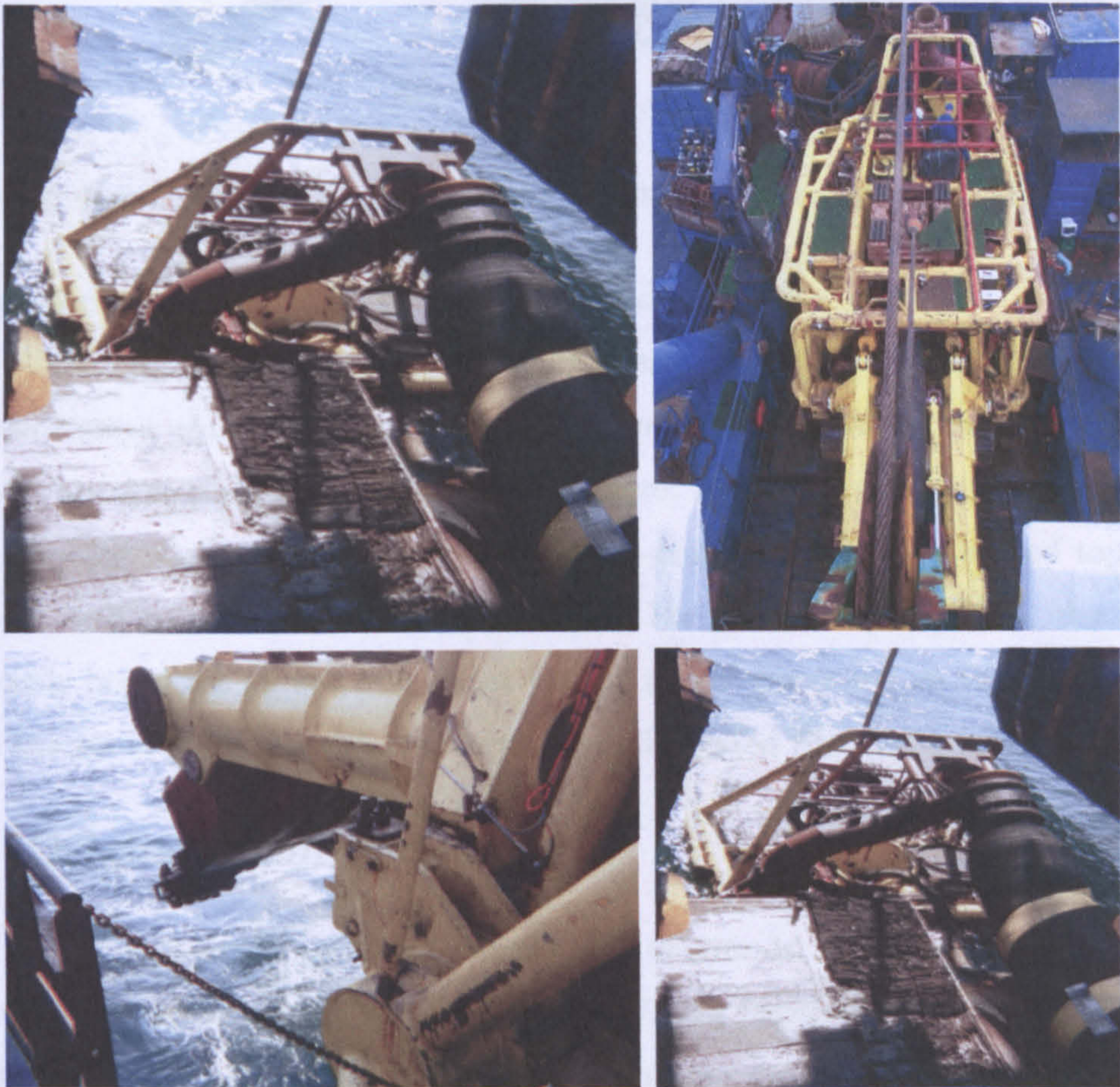
Figure 10.3: Photographs of the 180 tonne crawler being deployed
