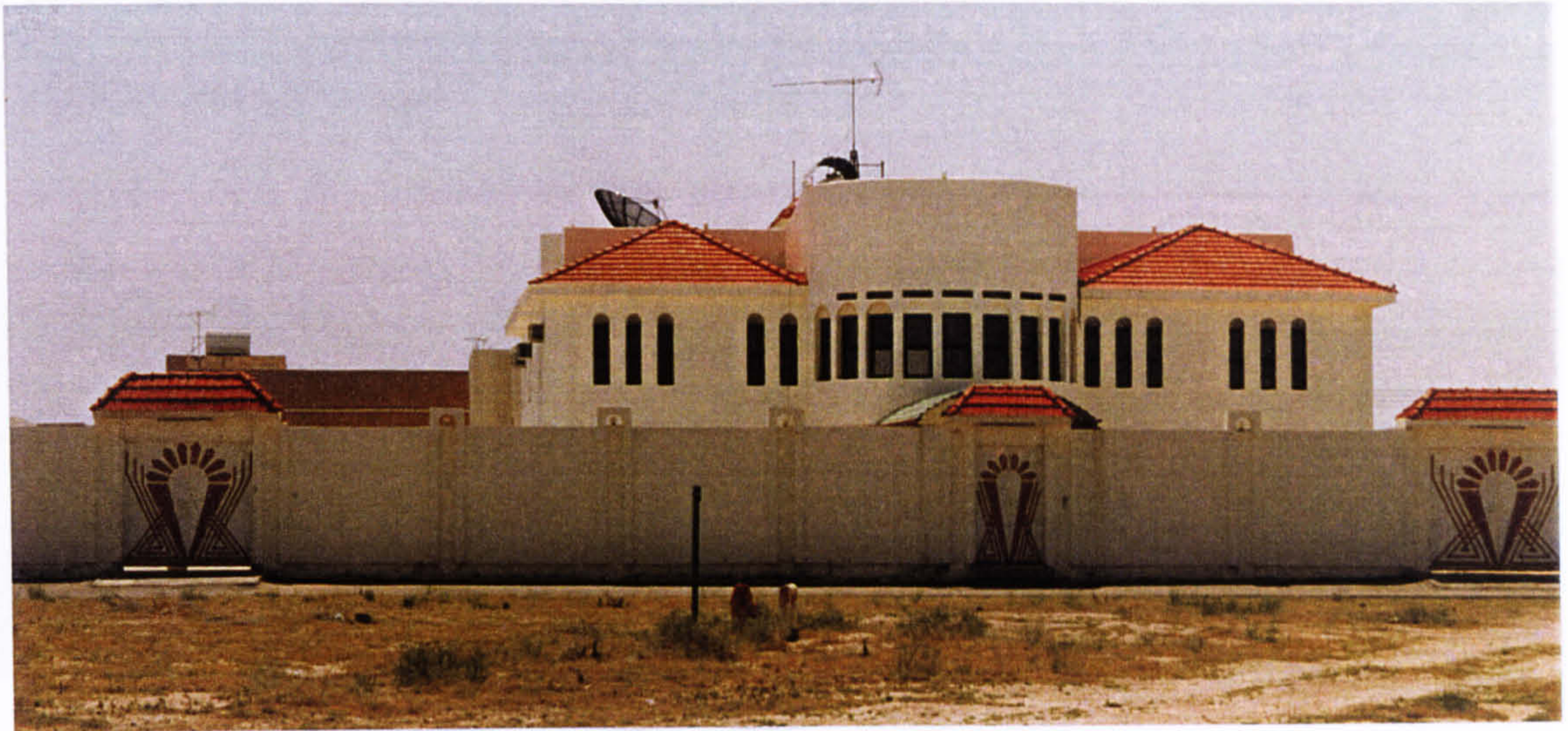
Figure 6.3. 1 A modern villa, showing a satellite dish in the roof
