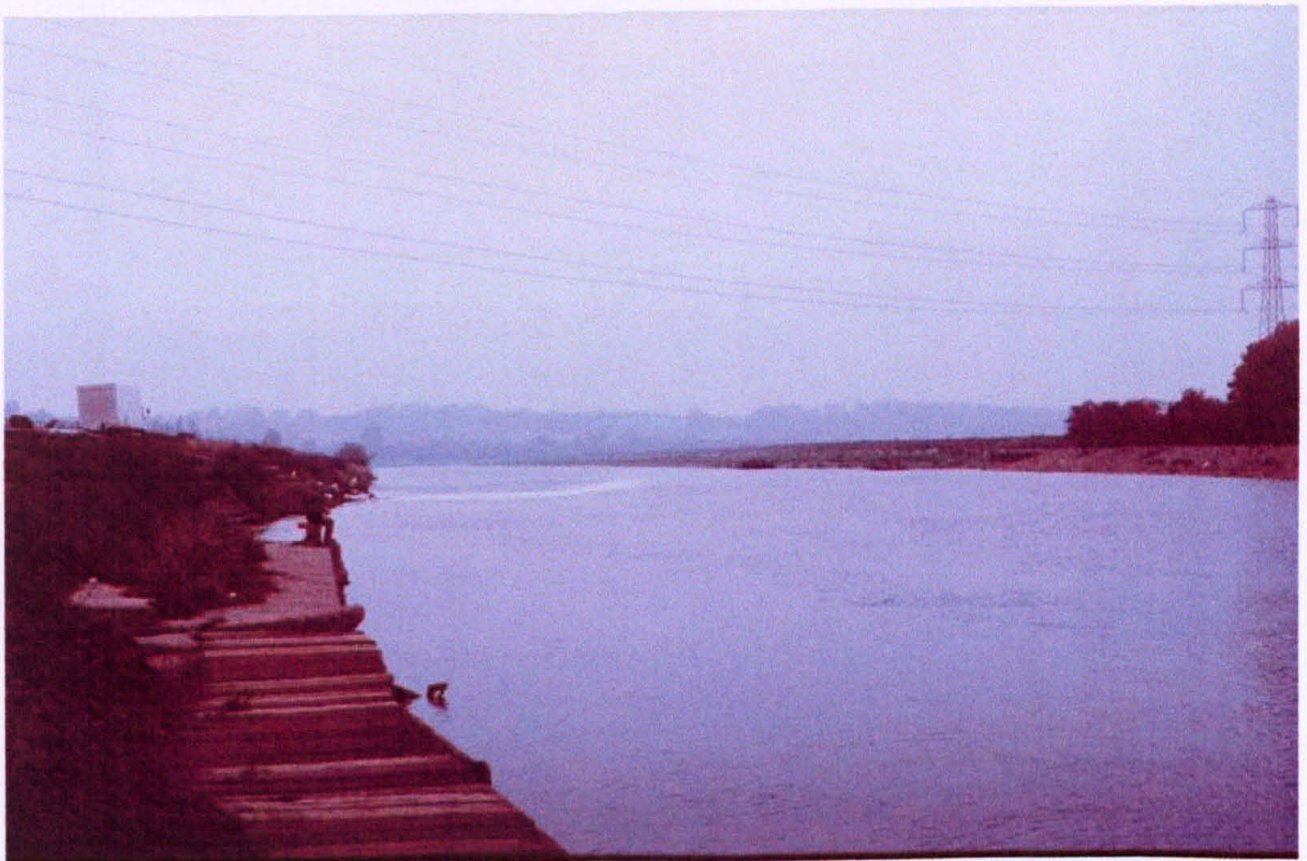
Plate 5.4 Stoke Bardolph sewage treatment works outfall, River Trent, viewed from further upstream.
