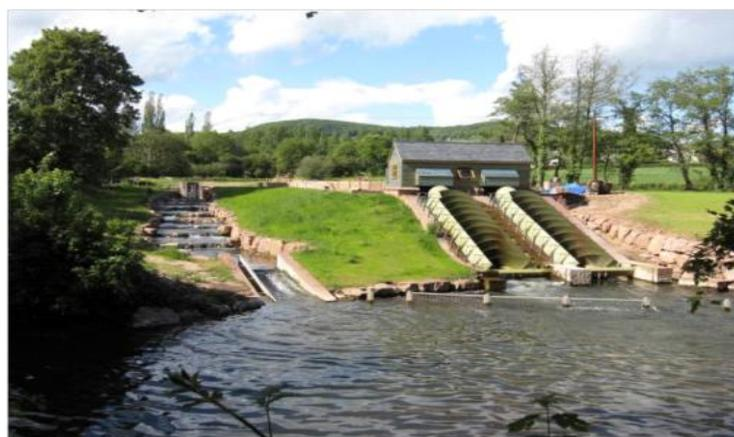
Figure 2.7 Archimedean hydropower turbine on a weir structure (photo courtesy J. Aldrick).
