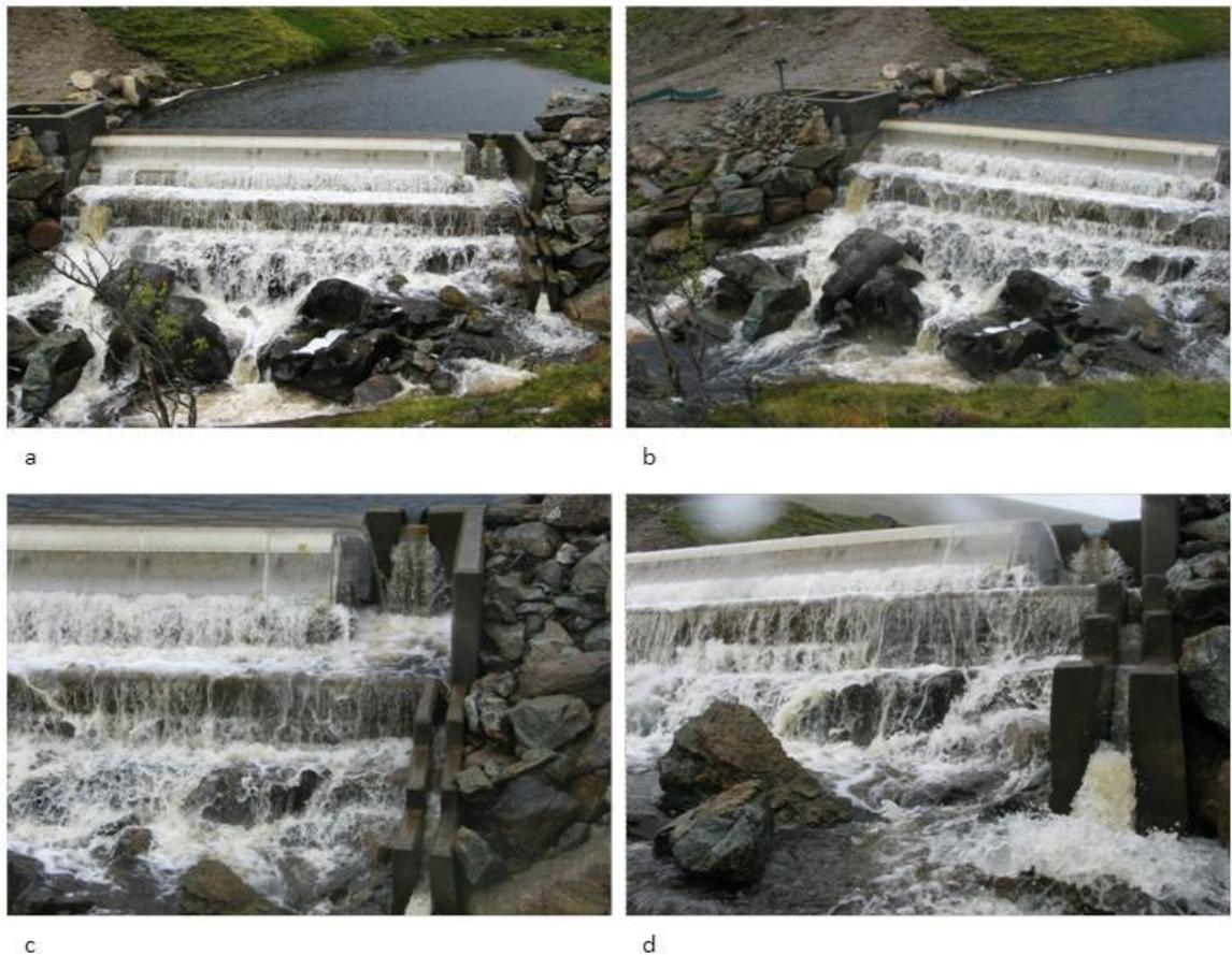
Figure 7.1 Fish pass constructed at Allt Gleann Da-Eig hydropower scheme. Photographs were taken September 2011.
