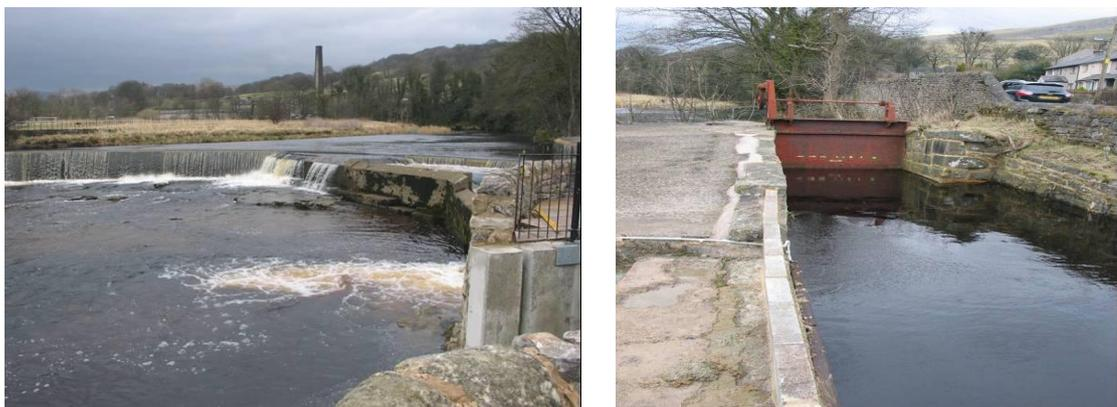
Figure 2.5 Existing weir on River Ribble, Settle (left), originally used to divert water to a mill via a mill leat (right), now used for diversion to a hydropower turbine.
