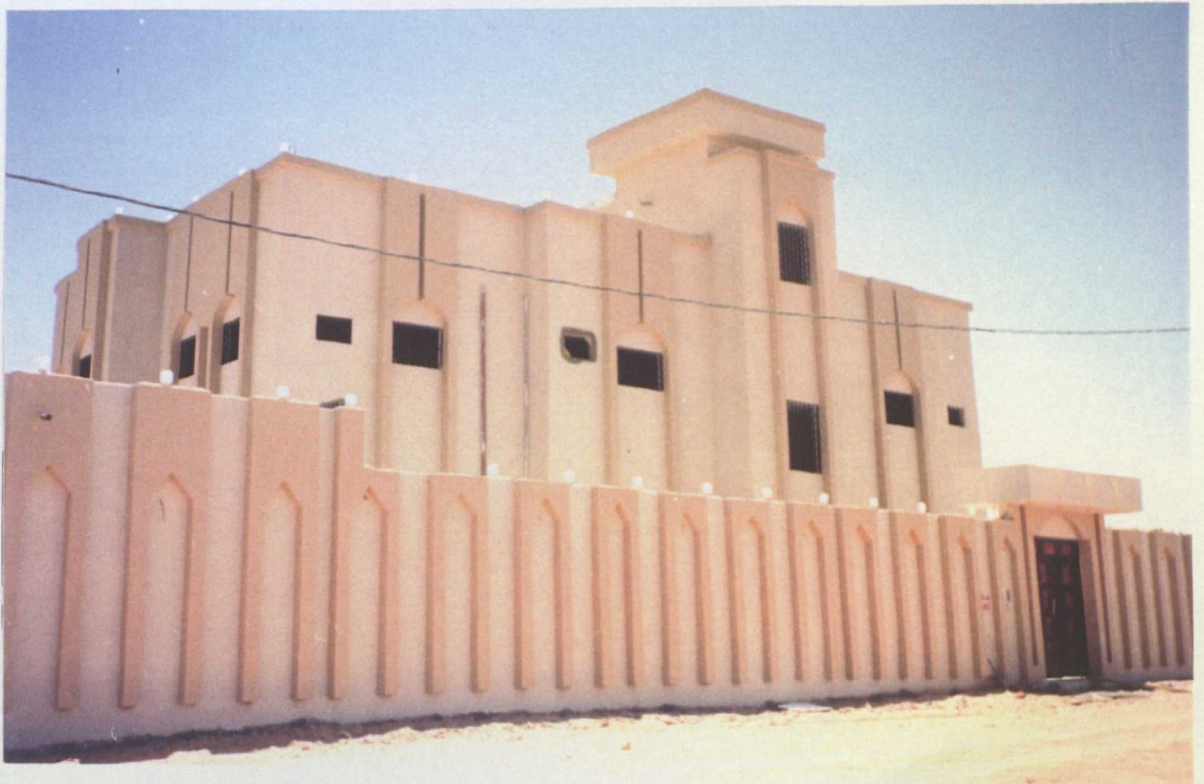
b) A Modern House in Hwylan built partly with a loan from the REDF
