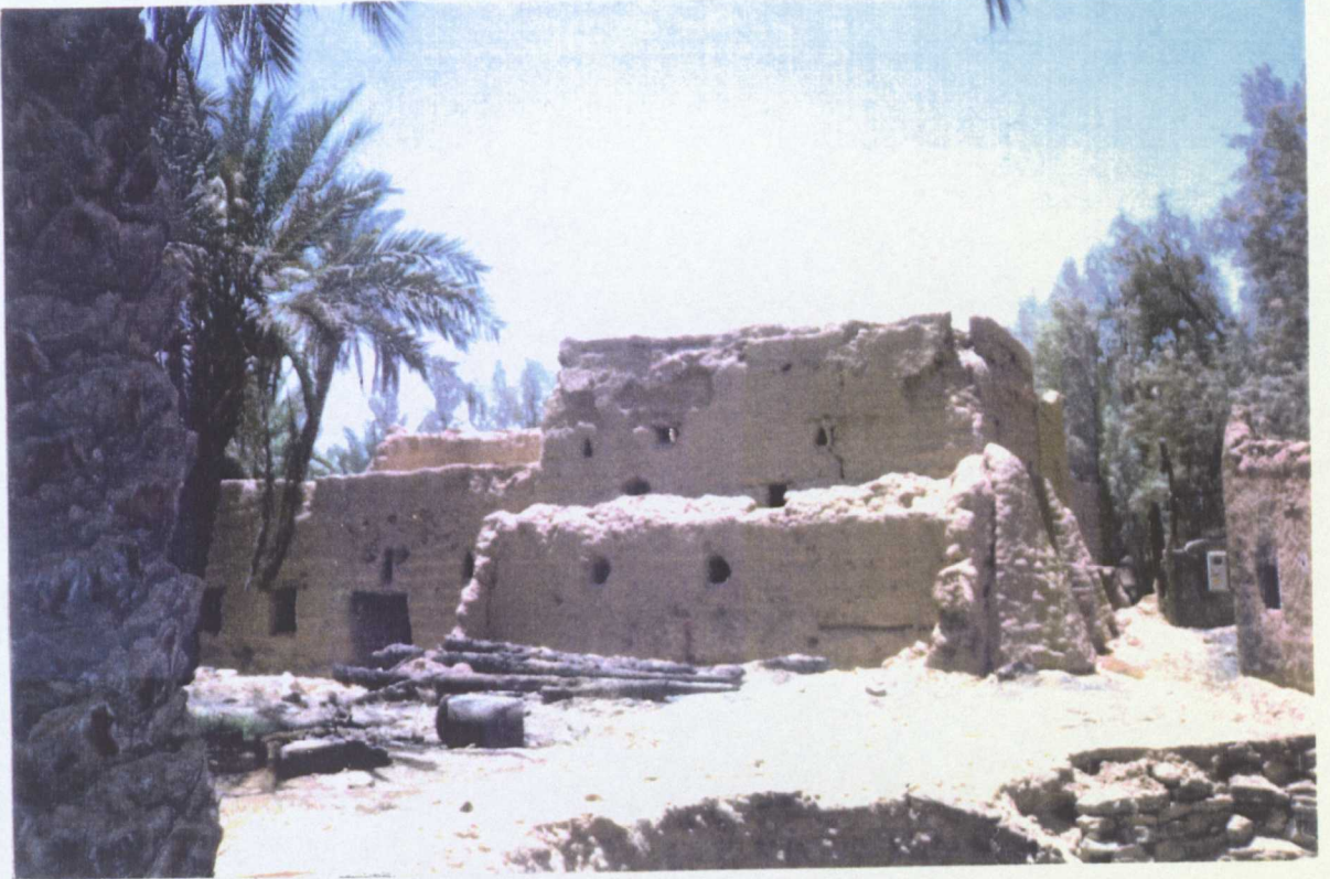
a) Abandoned Mud Houses in Disrepair in Hwylan
