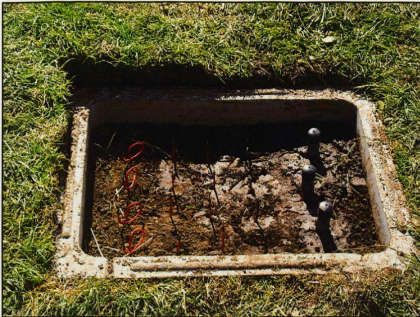
Figure 2.6: Monitoring point at Hatfield Moor showing piezometers and redox probes in situ .
