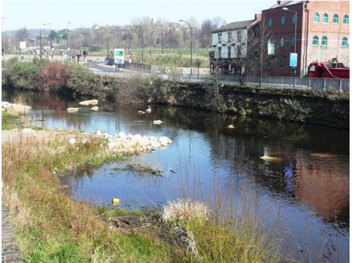
Figure 4.13. A triangular 'flow deflector' at Nursery Street, River Don (source: Environment Agency 2009).
