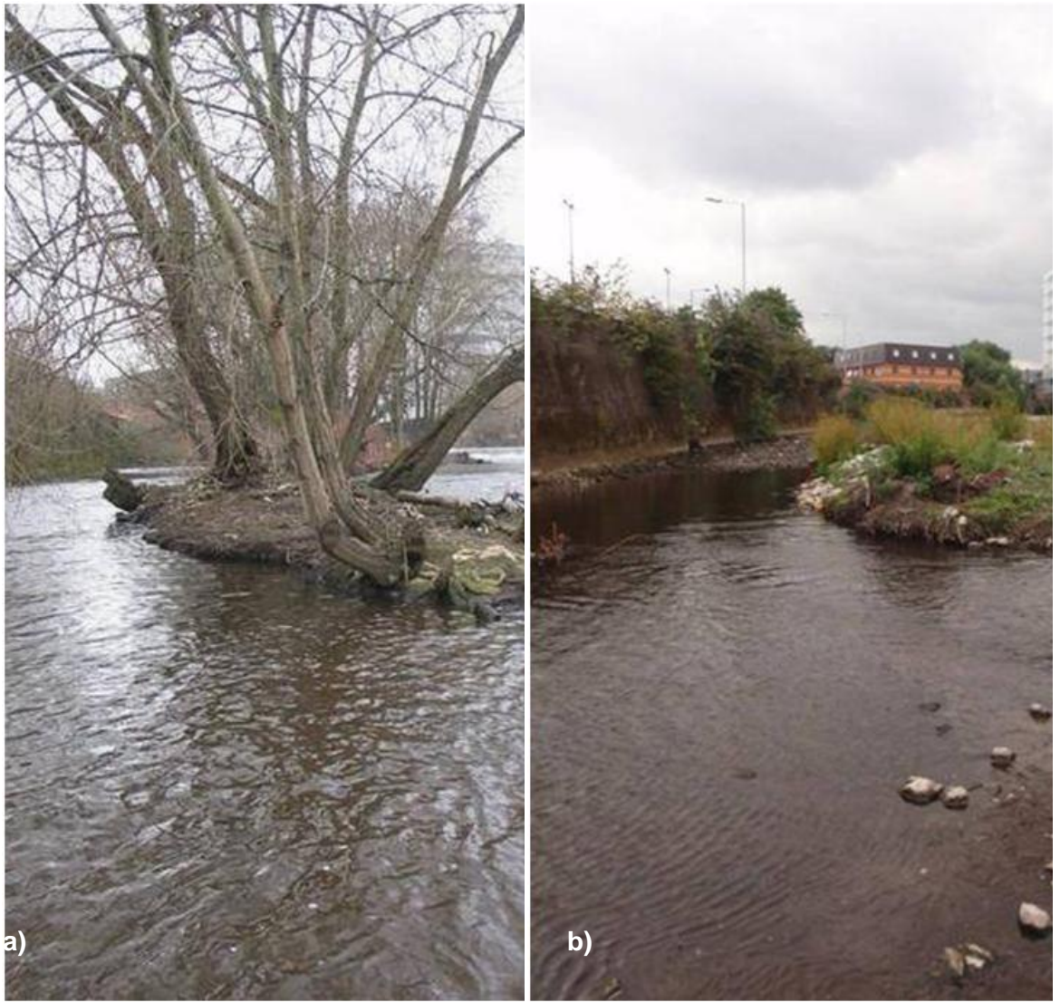
Figure 4.17. Photograph of Effingham Street before (a) and after (b) flood mitigation and rehabilitation works.
