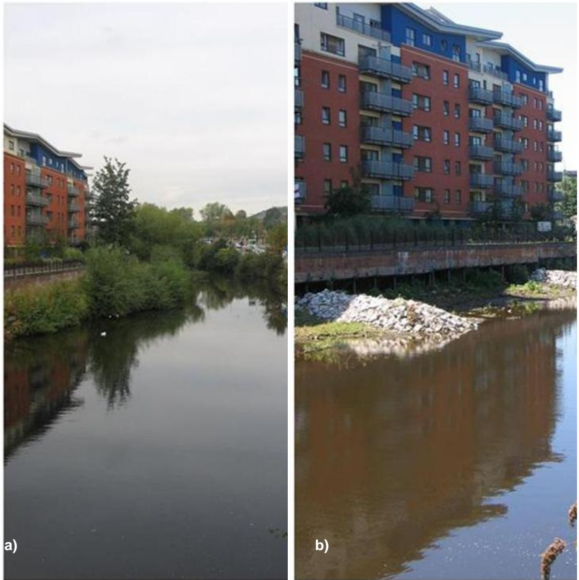
Figure 4.14. Photograph of Nursery Street before (a) and after (b) flood mitigation and rehabilitation works.
