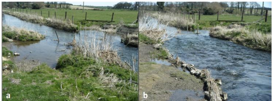
Figure 3.31. The River Stiffkey a) before and b) after channel narrowing and gravel introduction.
