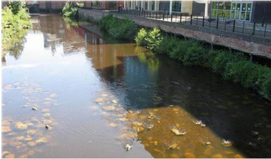
Figure 4.15. Rock riffle (a) at Nursery Street, River Don, downstream of the arched pedestrian bridge.
