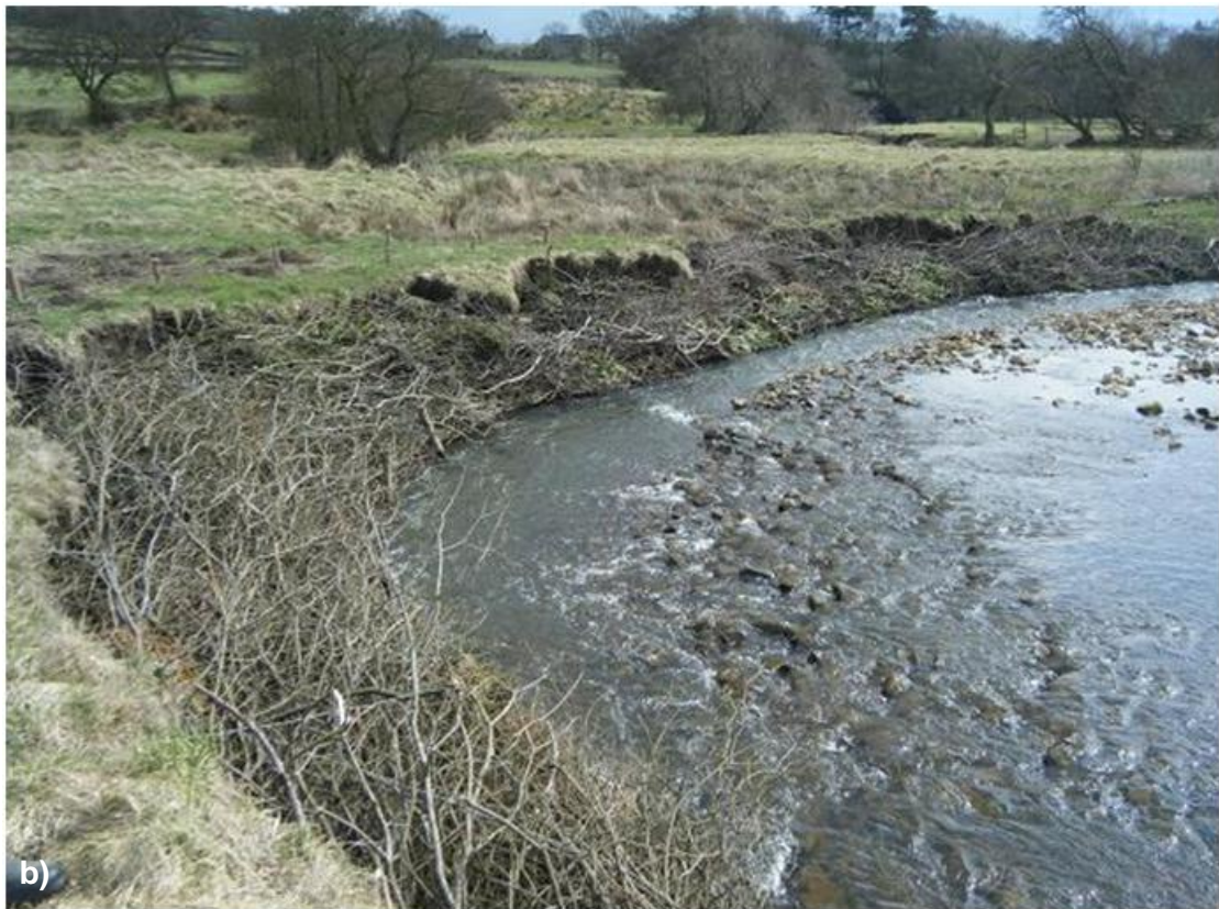
Figure 3.14. River Manifold a) bank erosion b) brush revetment as a measure to reduce bank erosion.
