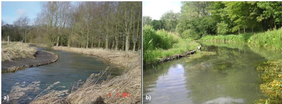
Figure 3.7. Channel narrowing on Lowthorpe Beck a) immediately after works February 2011 b) established margin July 2011.
