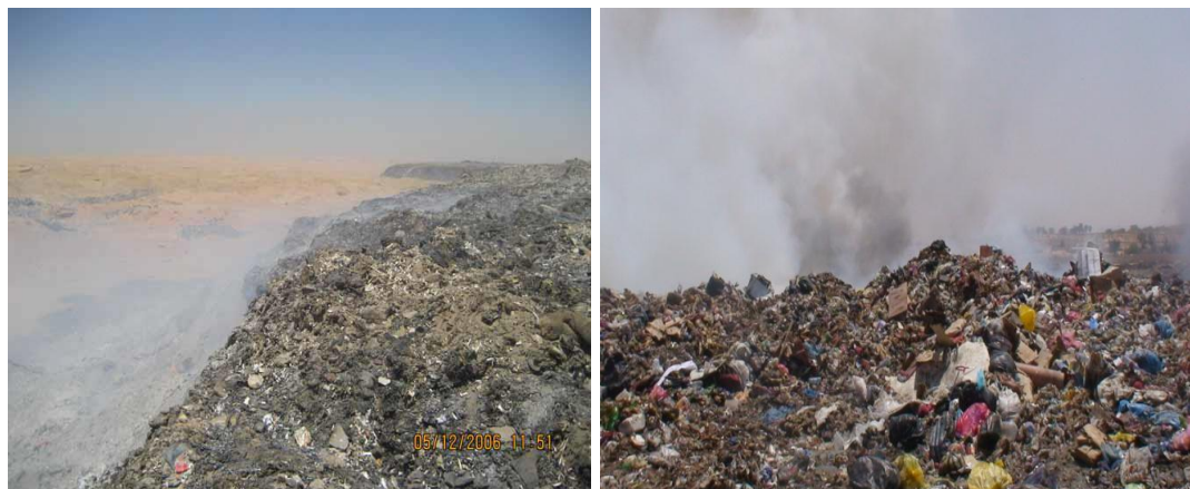
Figure 5-17: Landfill fire at managed dump, Sidi Al-Siah landfill
