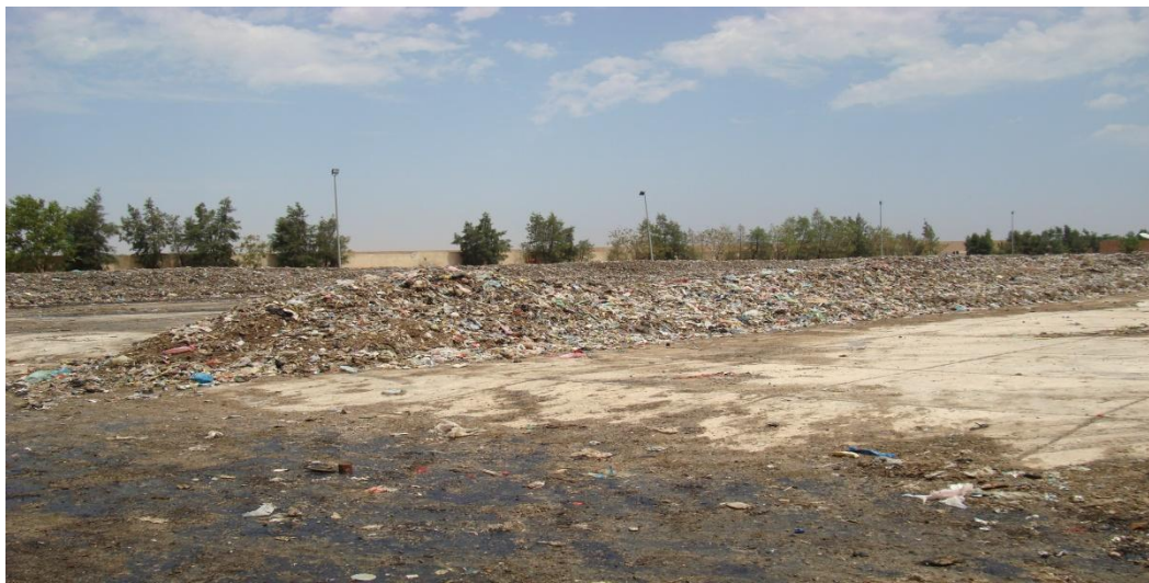
Figure 5-11: Release of leachate in Sidi Al-saih composting plant
