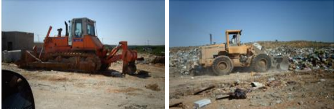
Figure 5-16: Equipment used to settle and compact waste at Alazizia landfill
