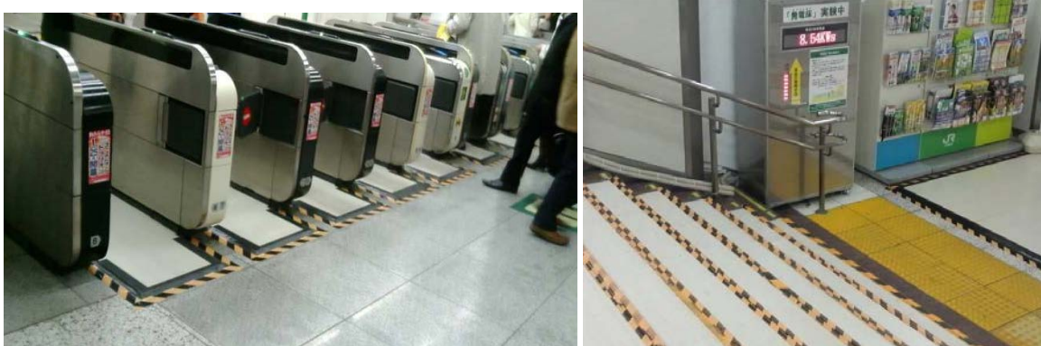
Figure 2-4 Energy Harvesting Ticket gate and staircase, Tokyo [90], [91]
