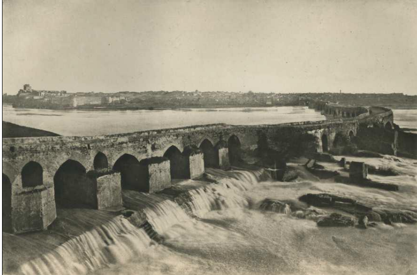
Figure 4.11 The Band-e Qaisar at Shushtar in 1884 AD, showing how it raised water levels upstream of it to feed the Masrukan and Darian canals (From Dieulafoy, 1885)
