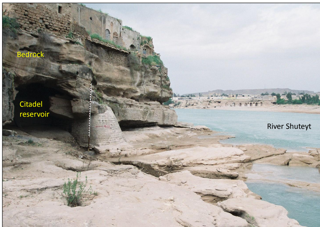
Figure 4.12 Citadel reservoir beneath the Salasel Castle in Shushtar (location of Salasel Castle shown on Fig. 4.13, looking W, staff divided into 10 cm graduations) This photograph of March 2002 AD shows the ancient citadel reservoir was not being filled by water from the River Shuteyt, even with spring seasonal high river water levels
