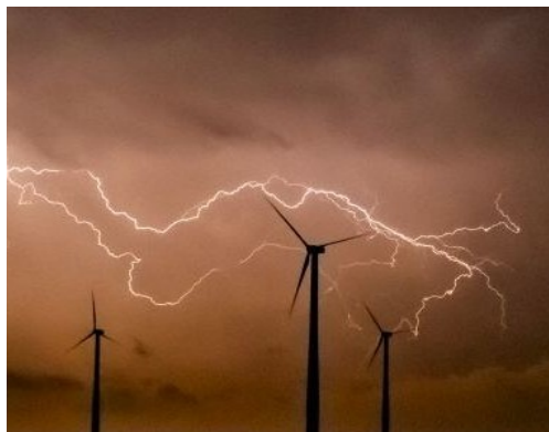
Figure 4-1 Lightning strike on wind turbine
