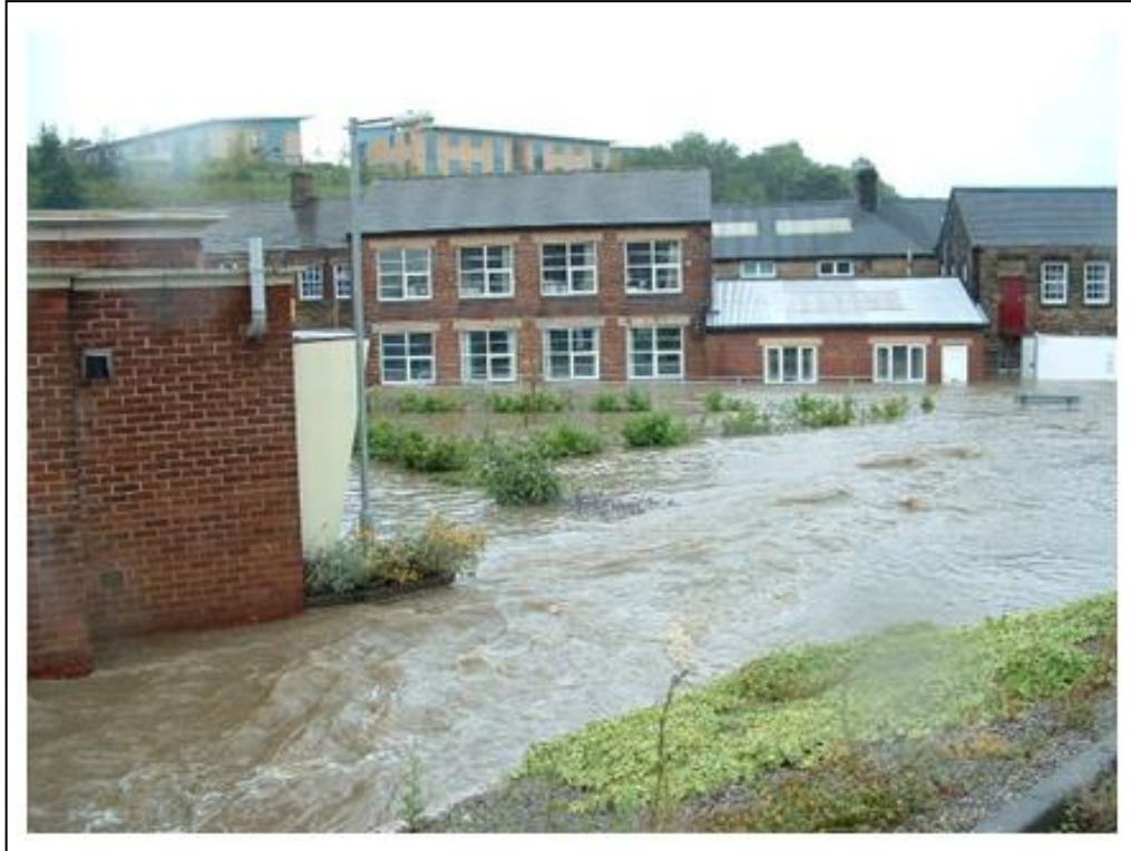
Figure 5.1: Flooding of the 16 acre business enterprise park owned by Company R
