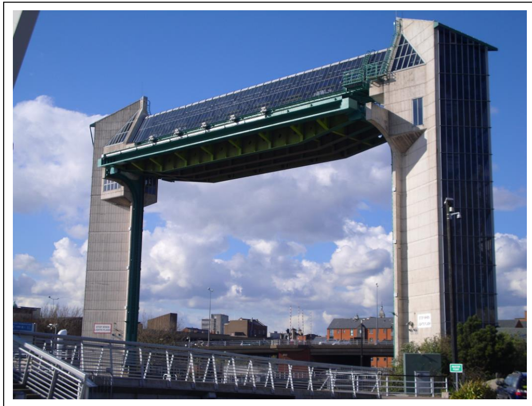
Figure 6.1: Hull Tidal Surge Barrier (Original Photograph)
