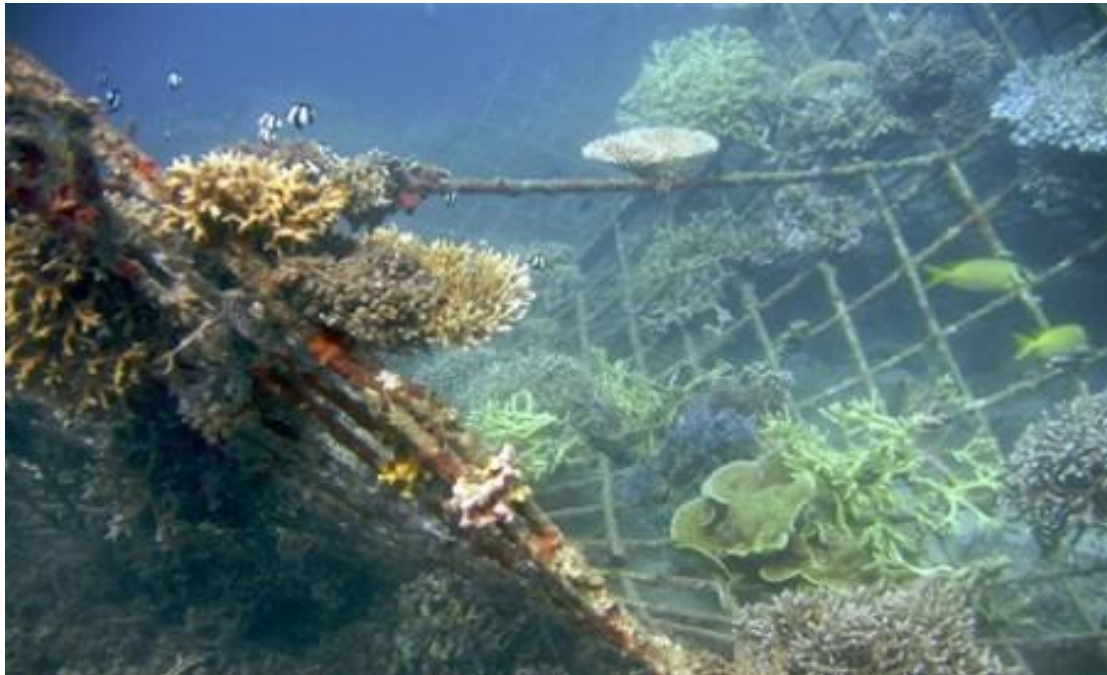
Figure 1.2 Biorock reef. Tetrahedron structure 5 years after installation consisting of accreted Biorock and developing coral nubbins (van Treeck and Eisinger, 2008).
