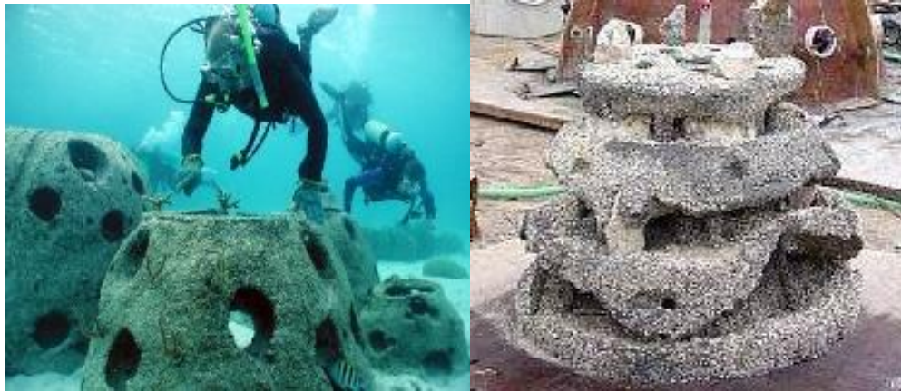
Figure 1.4 Examples of Reef Balls™. Standard Reef Balls™ (left) in three sizes and a layer cake Reef Ball™ ( www.reefball.org ).
