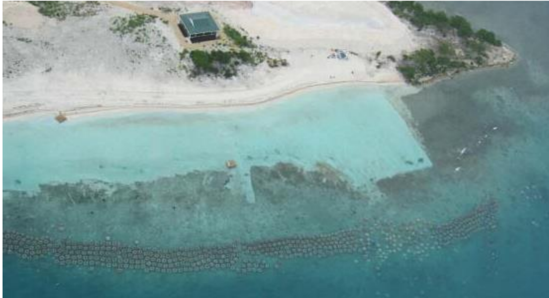
Figure 1.5 Aerial photograph of a 5-row Reef Ball™ breakwater structure in Antigua. Gaps and special areas have been incorporated into the design to accommodate divers and snorkellers (Harris, 2006).
