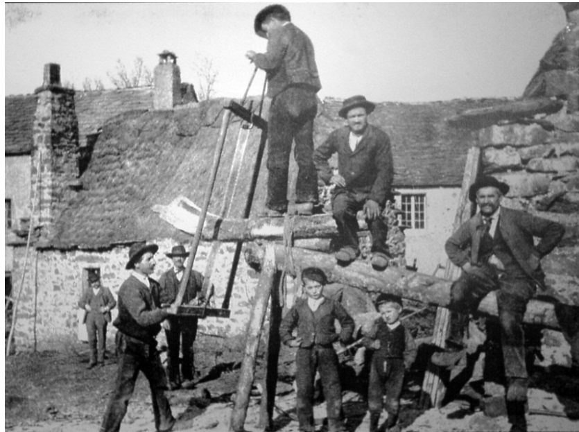
Fig. 1.10. A postcard of unknown date from the French Alps shows how a tree is sawn to make an alphorn.
