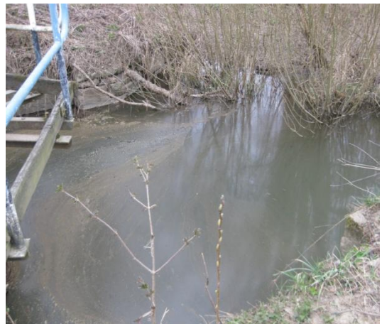
f) Disused lock of Howsham Mill
