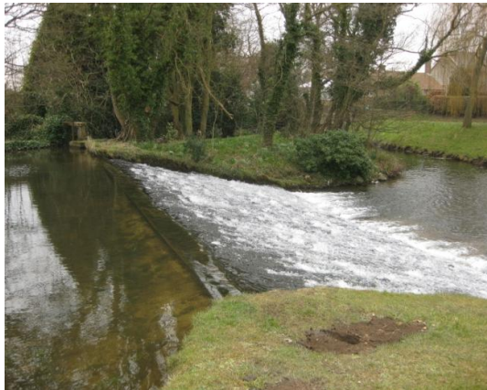
c) West Ayton weir and sluice gate (fisheries site 7)
