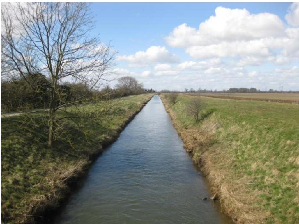
Figure 3.7 Heavily channelised section of the River Derwent with very limited riparian habitat (looking west from Brompton Bridge, downstream)
