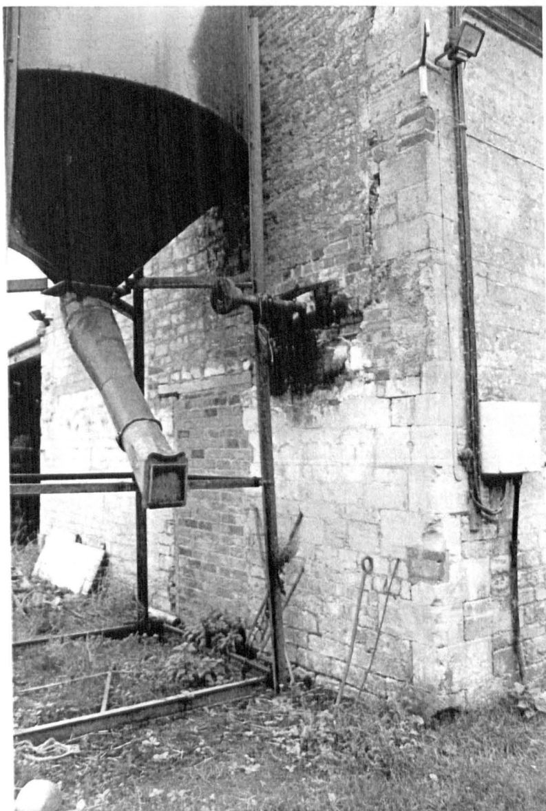
Plate 81 Remains of pulley wheel on exterior of barn wall, Hall Farm, South Rauceby
