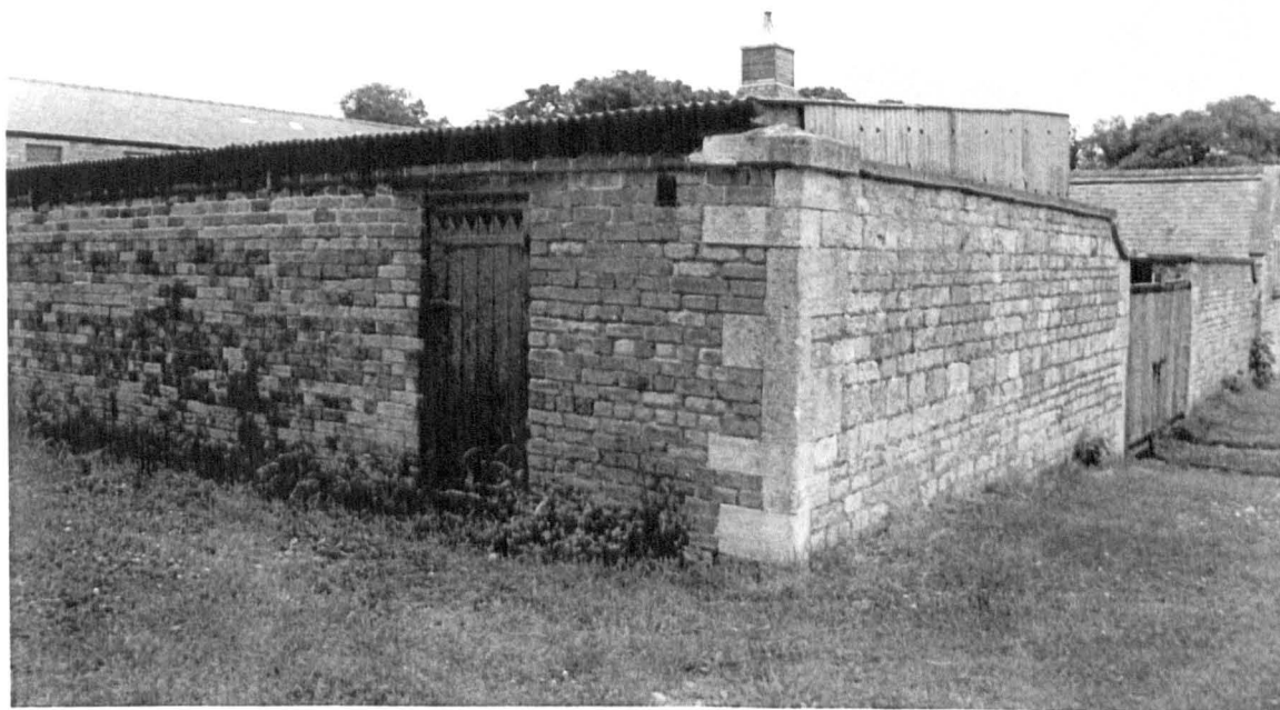
Plate 140 Stone façade and brick side walls of the crewyard at Grange Farm, Little Ponton
