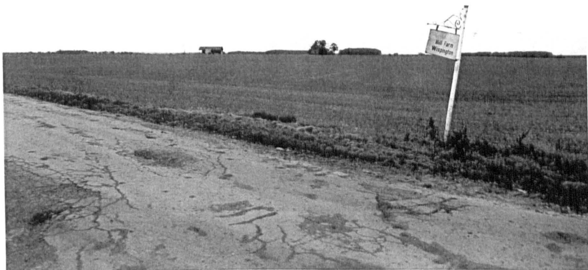
Plate 65 Farm name and road laid with rubble from the demolished farm buildings, Hill Farm, Wispington
