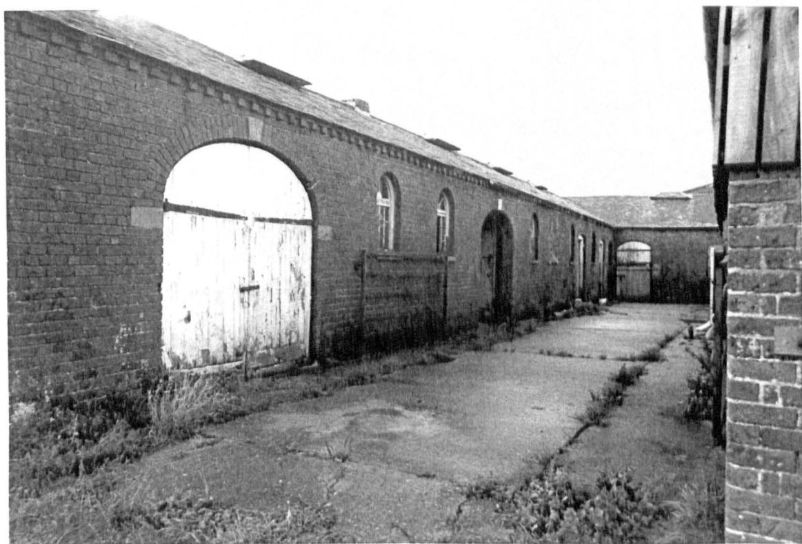
Plate 114 Brick arched windows and doors, stable range, Newstead Farm, Stixwould
