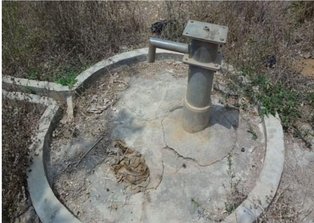
Figure 4.1 One of the non-functional bore holes available in Yekemi village Source: Fieldwork 2012
