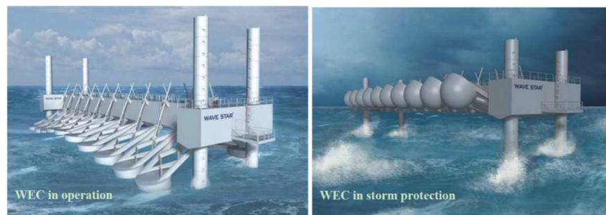
Fig. 2.4 Wavestar in operation and protection modes (Kramer et al., 2011).
