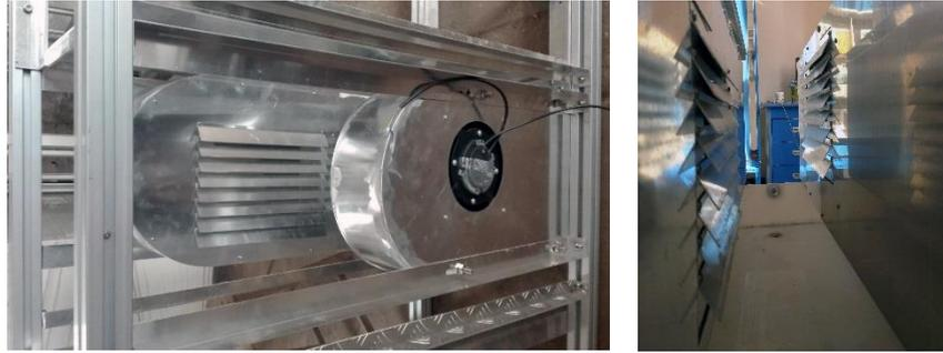
**Fig. 4-42: Louvres on the fan housing.**
