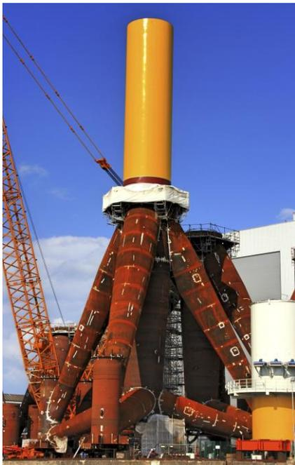
**Figure 2-31 – Tripod Foundation**
