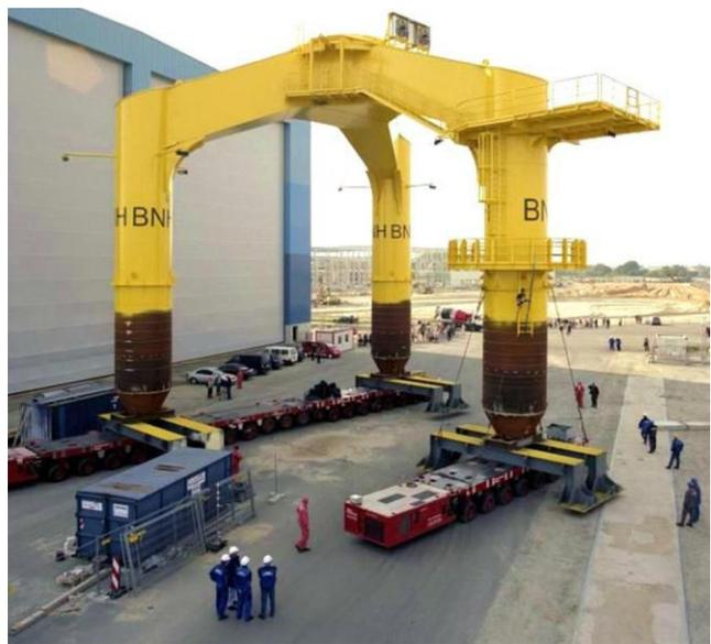
**Figure 2-32 – Tri-pile Foundation (Brickwell, 2012)**
