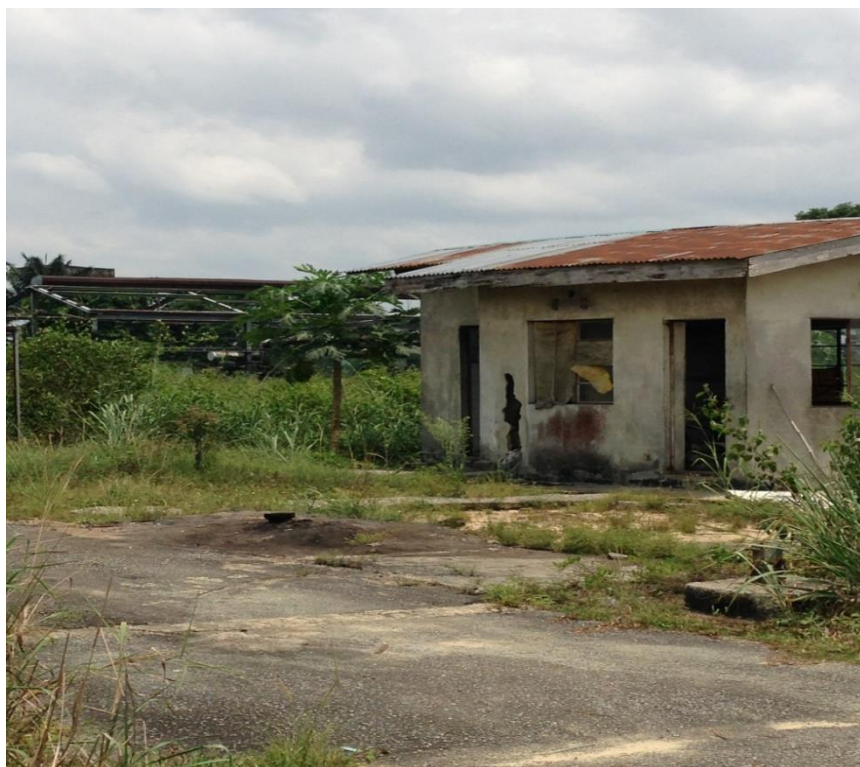
Figure 19: Abandoned School Project, Eleme Village
