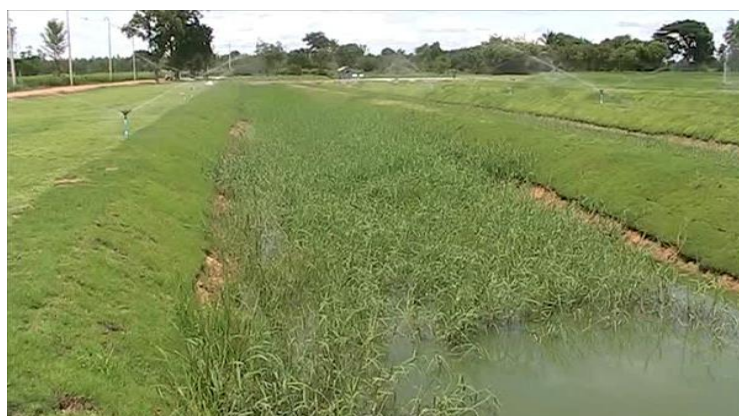
Figure 25 Grass filtration (Source: author)
