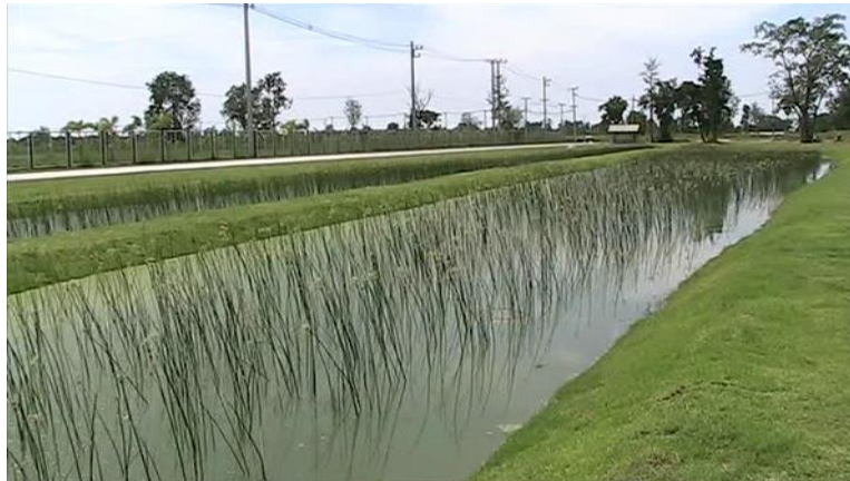
Figure 24 Constructed wetland (Source: author)
