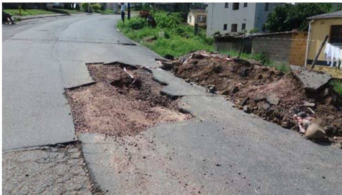
Figure 4.6: A road damaged after an extreme rainfall event in Lamontville Central (Source: Author's own)
