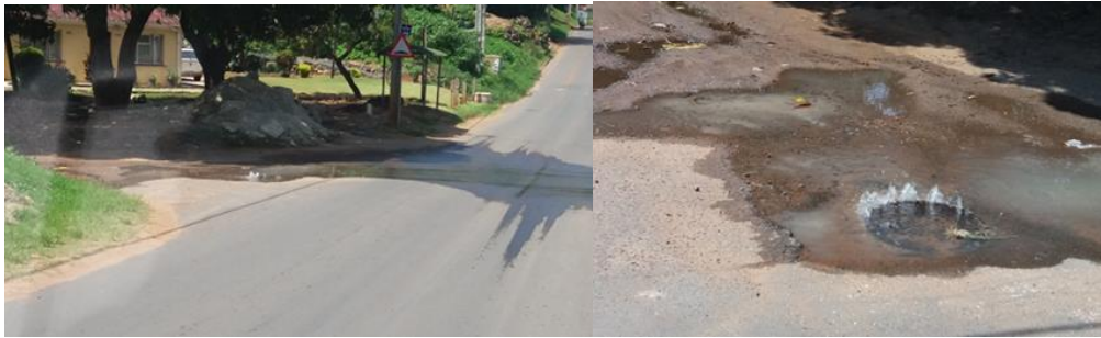
Figure 4.7: Road damaged by burst sewerage pipe in Lamontville Central (Source: Author's own)
