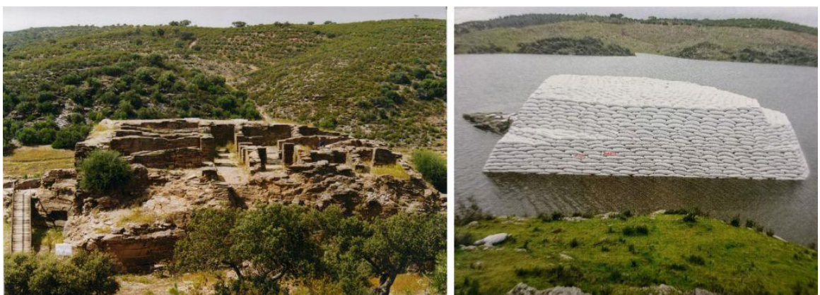
Figure A.4 Castle of Lousa before submersion (left) and protected and ready for submersion (right) (source: http://blogueequipa4itec.blogspot.co.uk ; EDIA).
