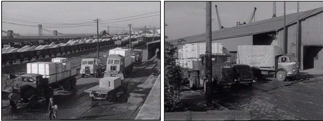
Figure 8: Still images taken from the British Transport Film's 'Berth 24' (1950) of road transport at the Hull docks. It is possible to see the narrow, cobbled roadways across the dock estate that were also obstructed by rail tracks.
