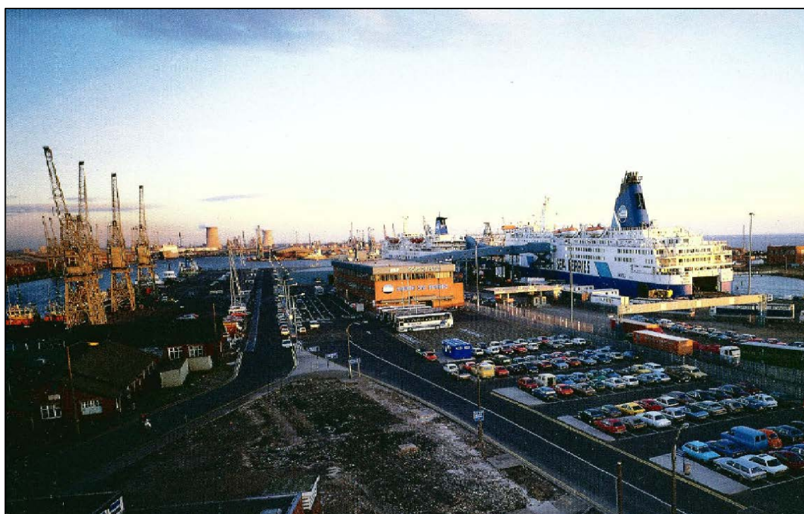
Figure 22: The Princess Margaret Terminal opened in 1987 at King George Dock epitomised ABP's intensive capital investment following privatisation. (Image from Associated British Ports, Port of Hull: Ro-Ro Services , 1989).
