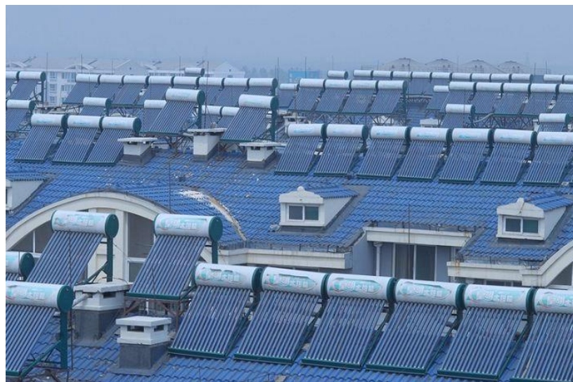
Figure 4.5 Evacuated tube SWH on building rooftops
