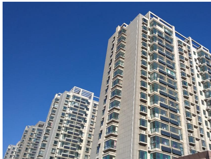
Figure 4.6 Flat-plate SWHs on high-rise buildings' balcony
