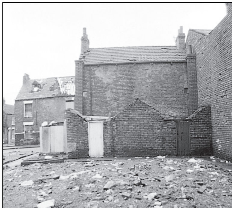
Figure 9. Demolition of Eton Street, south of Hessle Road, 1980. 84
