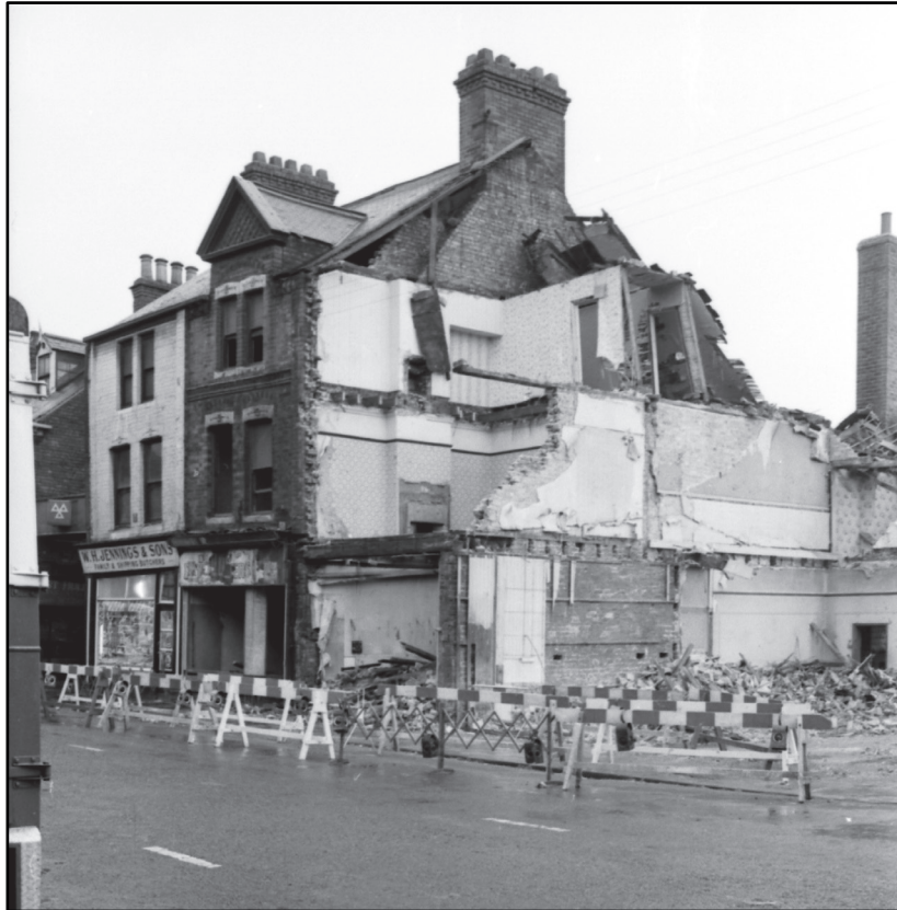
Figure 8. Demolition of 191-193 Hessle Road, 1966. 83
