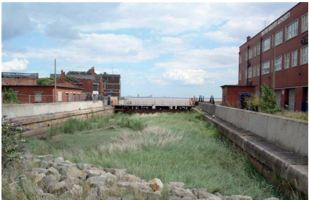
Figure 16. The silted lockpit looking out to the Humber. To the left a cluster of small offices and stores once typical of the Fish Dock. To the right, the larger office of the White Fish Authority stands on the bullnose. 54
