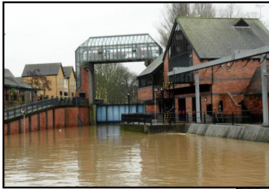
Foss pumping station and floodgate
