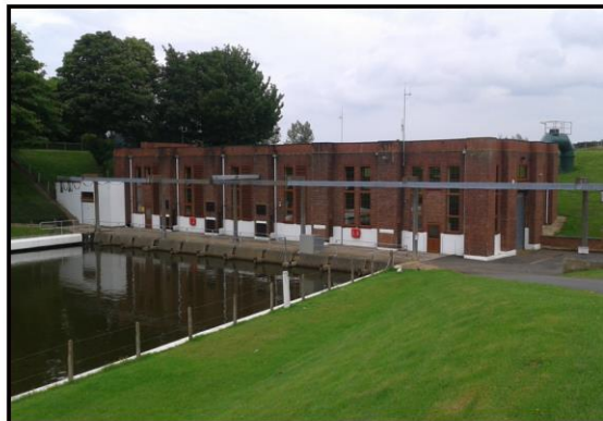
Tydd pumping station
