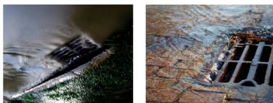
Partial Blocked (Classified as Fully Blocked) No Blockage (Classified as partial blocked)
