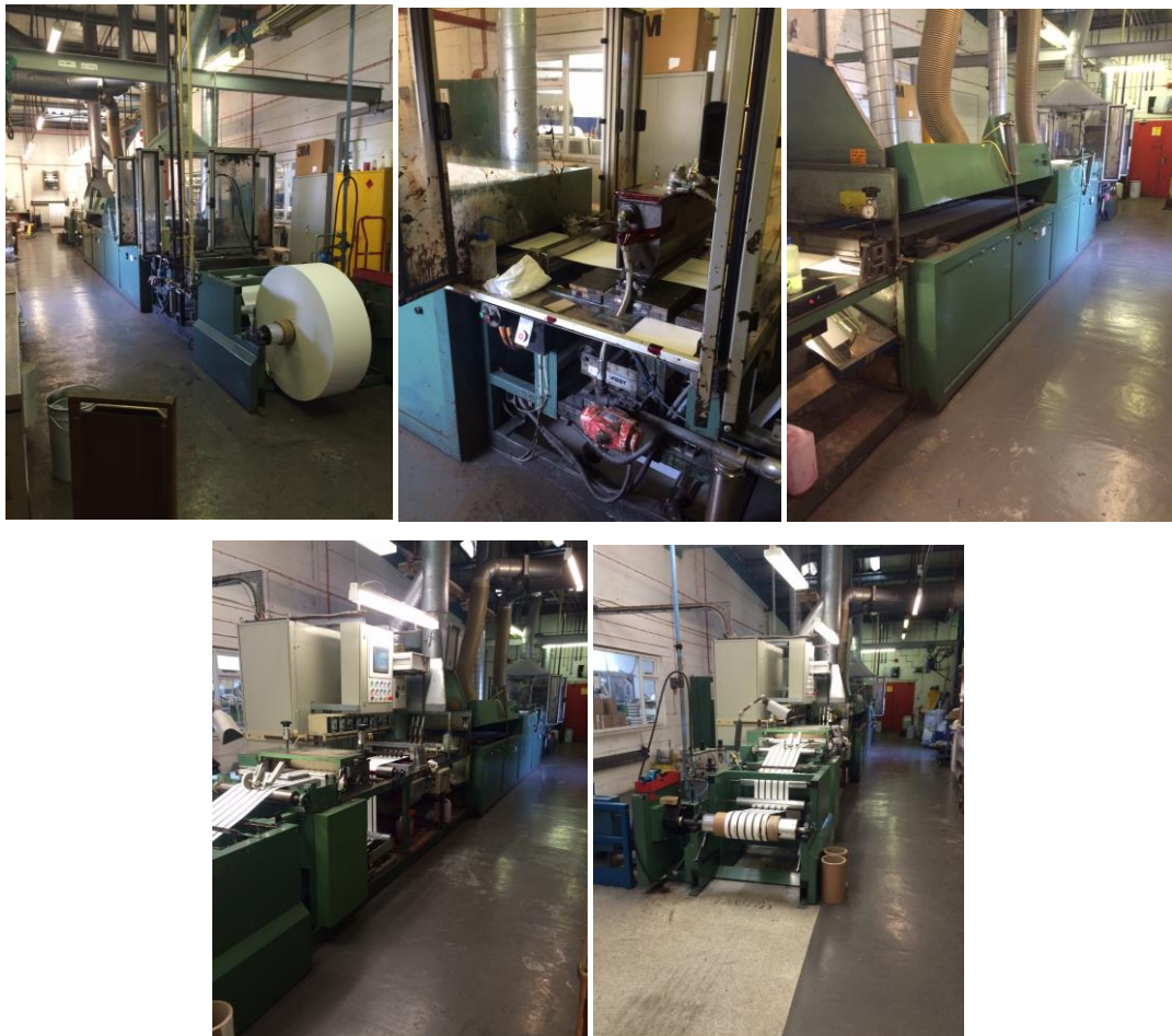
Figures 2.13 to 2.18: Photographs of the Magnacoater at BBP Hull.
