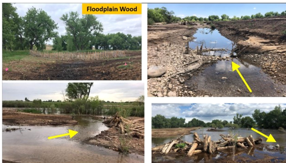
FIGURE 3 Examples of wood structures emplaced in the floodplain and channel. Yellow arrows indicate flow direction. Credit Johannes Beeby. [Color figure can be viewed at wileyonlinelibrary.com ]
