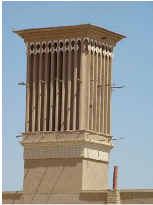
Figure 19 - A four-directional bagdir (wind catcher) in Yazd, Iran [137]
