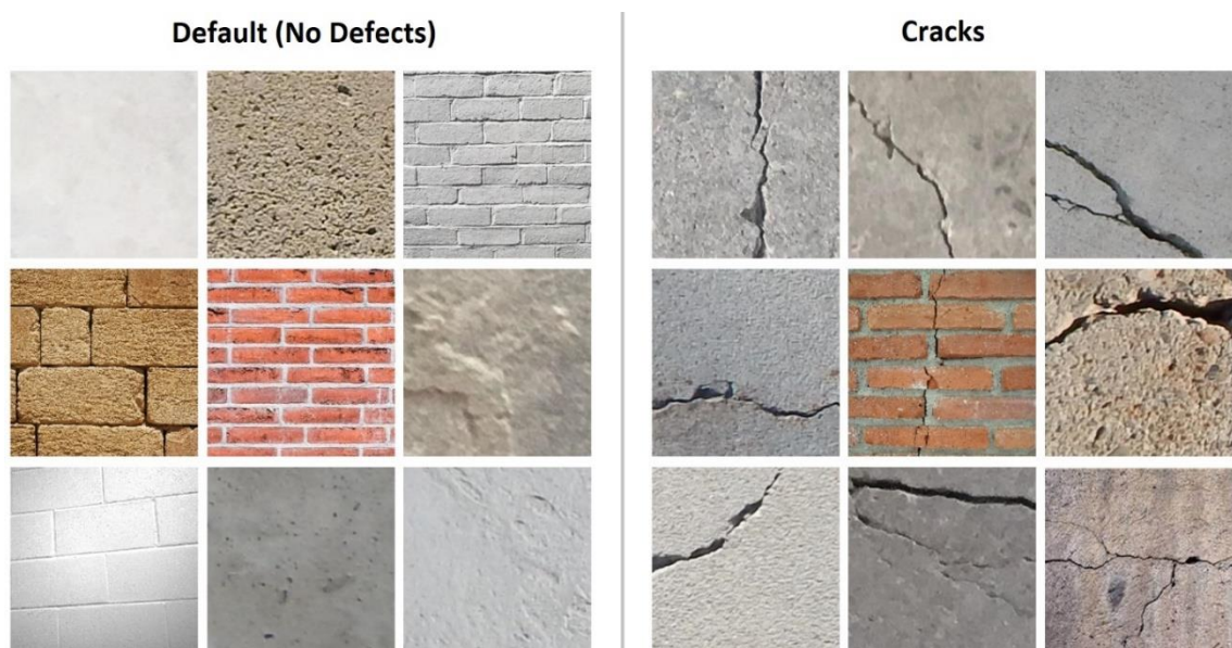
Figure 38 - Examples of training dataset for ‘default’ and ‘cracks’ in supervised model
