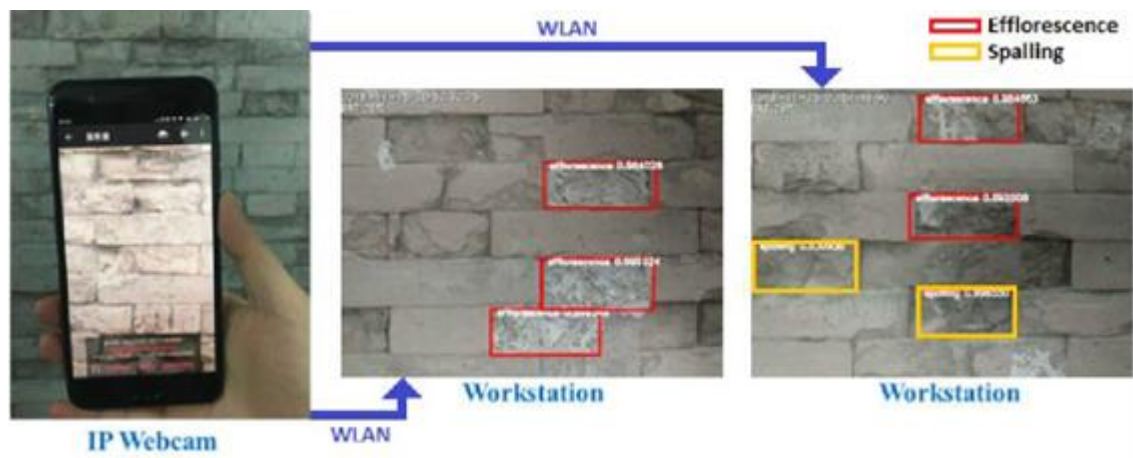
Figure 8 - Damages identified by CNN and shown in real-time via a smartphone [63]
