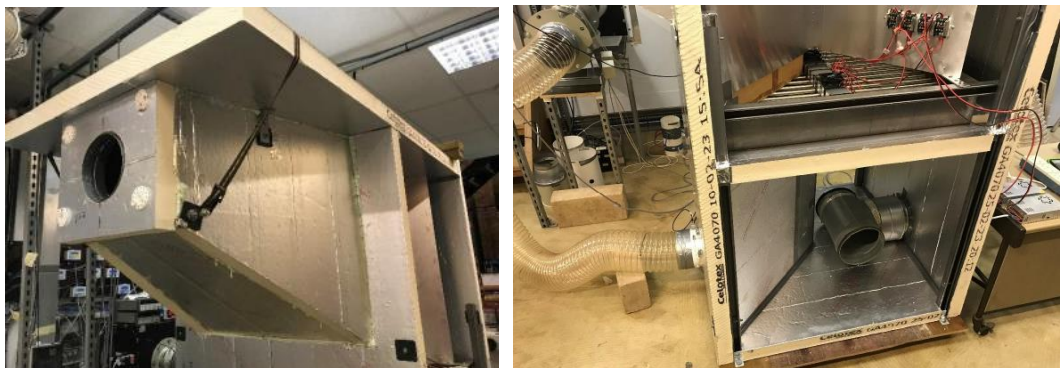
Figure 85 – Windward inlet for regulated air supply (left) and extract air system (right)
