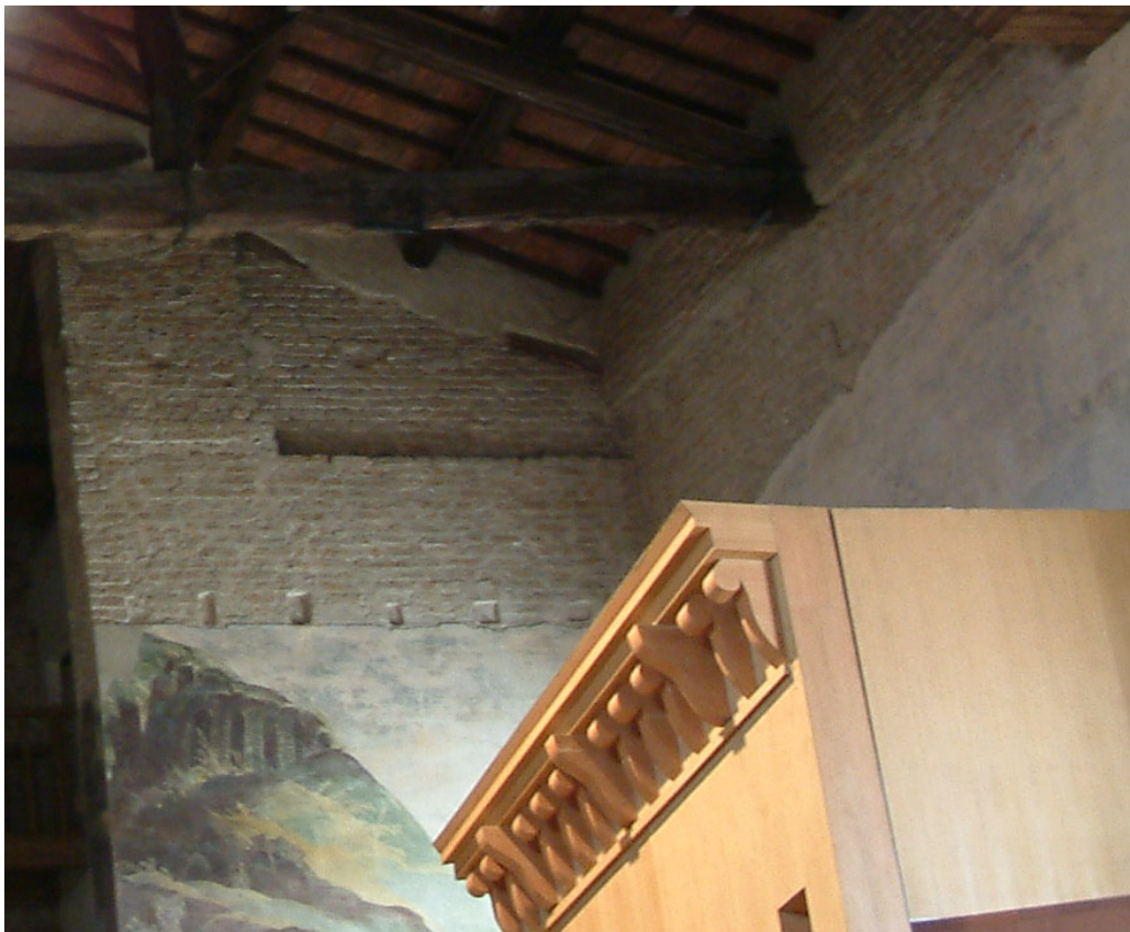
Figure 30. Roof Area Above the Stage (with modern reconstruction of stage setting)
