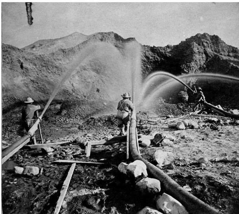
3. Hydraulic mining near French Corral, Nevada County, 1866. Courtesy of the Library of Congress, Washington, DC, Prints and Photographs Division, LOT 3544-50, no. 1404 [P&P].
