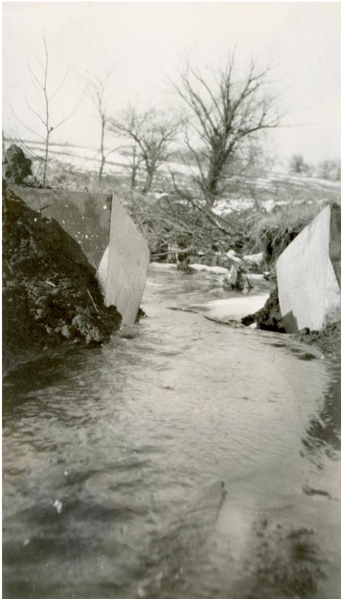
Figure 2: Flowing water from melted snow passing over gully control flume installed at the head of a gully in Ravine C near silt box C-10, Bethany Soil Erosion Experiment Station, March 24, 1932. A. T. Holman. National Archives and Records Administration (114-CS-7-88-12660).
