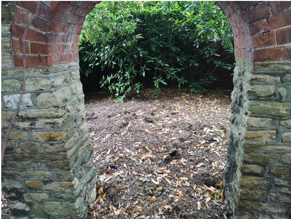
Figure 38 the purported "Roman" arch located in the grounds of a large house running between the Burrs Playing Field and The Burrs. Note not only modern brickwork completing the feature but the presence of modern mortar throughout, despite this there is possibly some argument that the stone itself is of Roman cut as the site lies within the boundary of the walled enclosure with any structure at this point likely to be truncated by the digging of foundations for the house.
