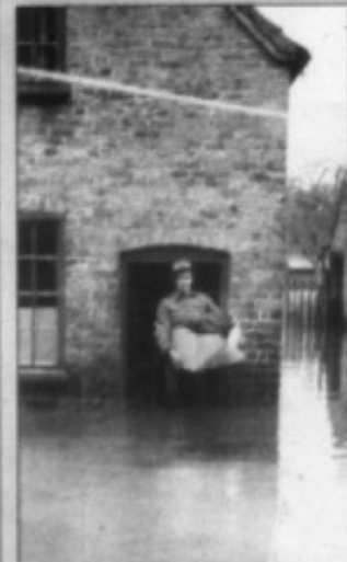
PICTURE NUMBER 6. In March 1949 Bishop Burton became flooded and the workmen's cottages had to be evacuated.
