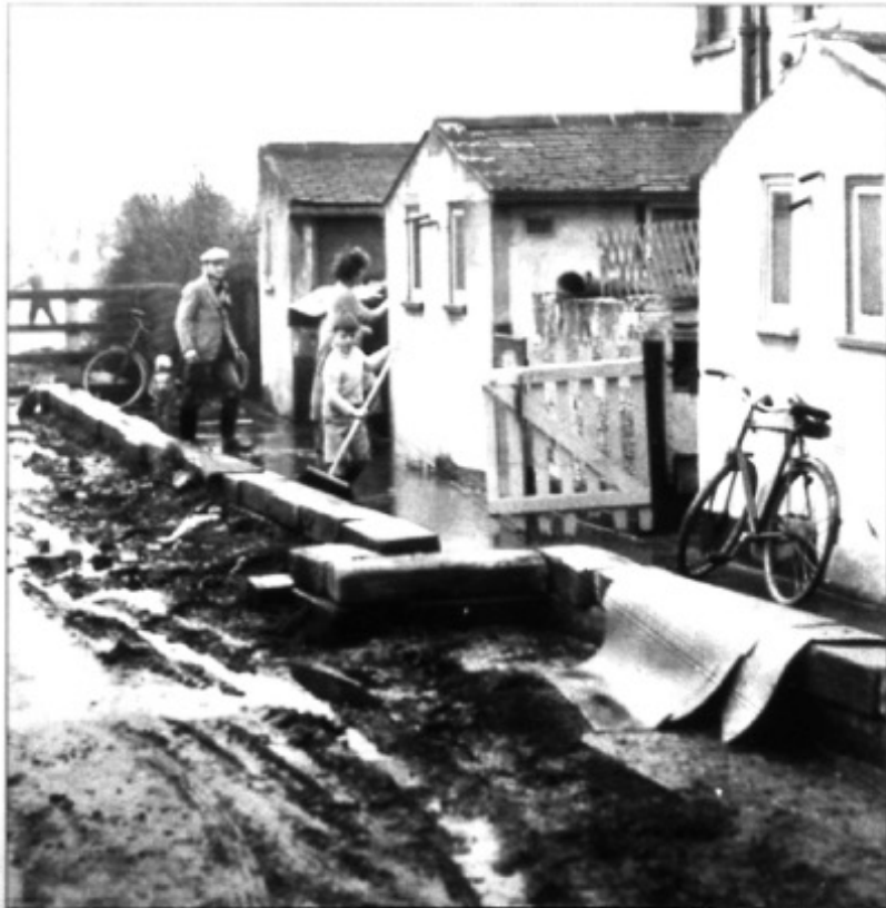
THE AFTERMATH: A scene of devastation at Brickyard Cottages, North Ferriby, as householders clear up after the flood.
