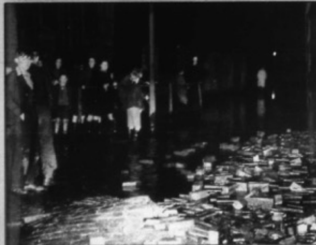
PICTURE FIVE. When the River Hull overflowed its banks in March 1949 it left a large amount of repair work to be done.
