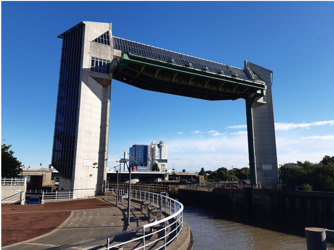
Figure 8. Flavia Manieri. The River Hull tidal surge barrier today. Sept 29, 2021.
