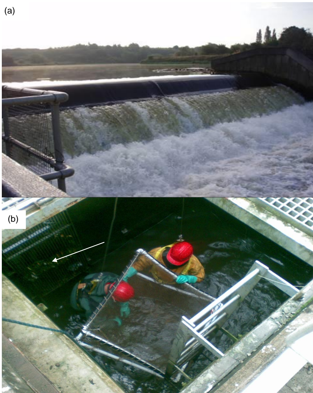
Figure 3.14 Photographs of Woolston weir; (a) the right hand flanking ogee weirs and (b) the trapping of salmon. Note the moveable pen-stock (closed) in the top left hand corner of the picture denoted by an arrow.
