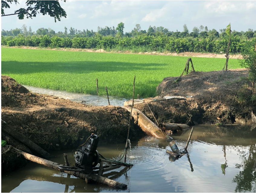
Figure 17: Pumping System in Ricefield taken by Researcher
