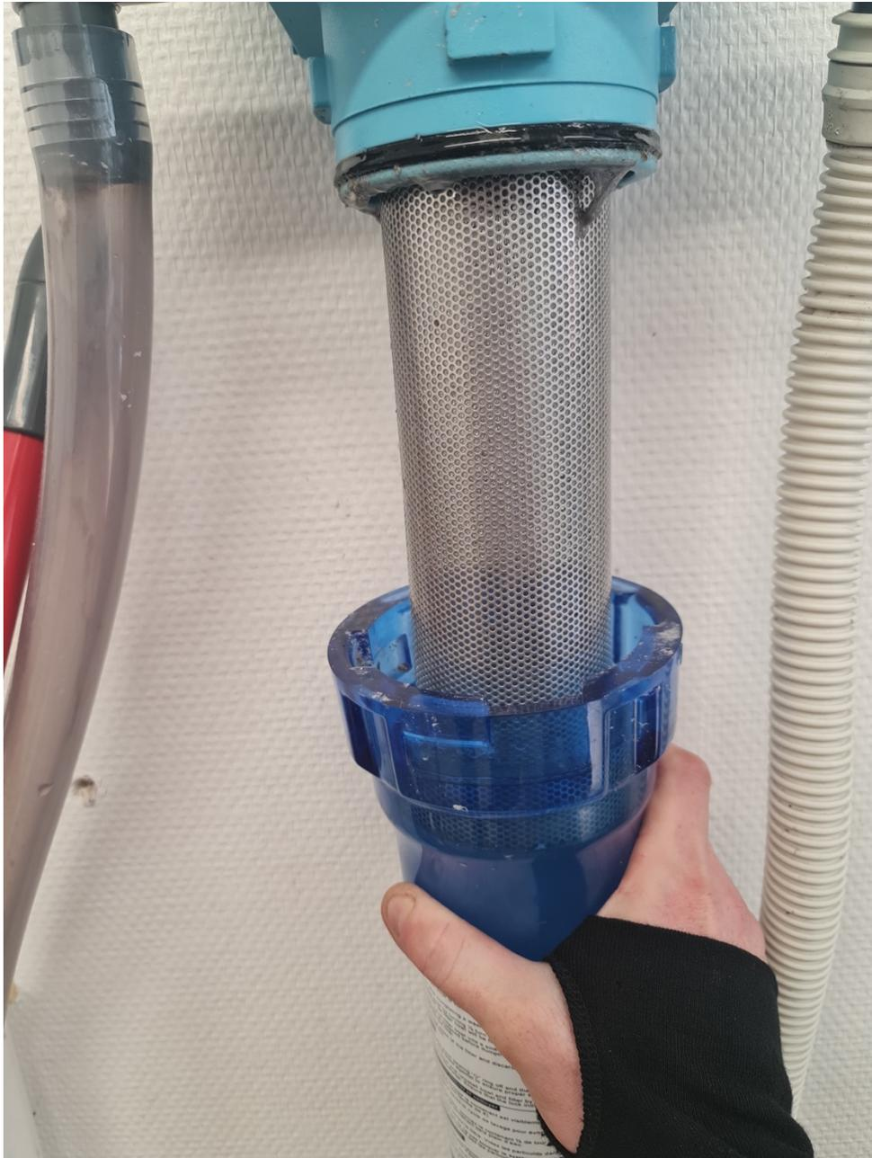
**Figure 1.6, an image of a filter attached to a washing machine at King Edward Point (KEP) Research Station, South Georgia, designed and fitted to catch large aggregations of microfibres and any other debris from washing clothes. Image provided by Joe Birdsey, British Antarctic Survey Maintenance Technician at KEP, 2021).**
