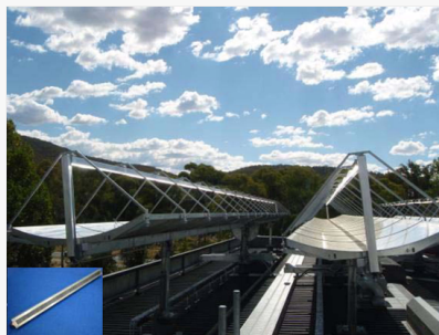
The CHAPS PV-Thermal hybrid concentrator on the roof of Bruce Hall (Canberra, Australia); and detail of the actively-cooled receiver [68].
