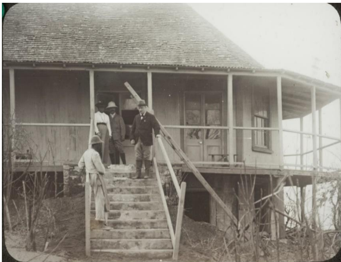
Figure 4.3. Untitled photograph taken by Tempest Anderson and held at the Yorkshire Museum (TA124). The house looks intact, the timber walls, doors, railings, steps and tile roofs appear relatively unscathed and not warped by heat. The window glass behind the woman and men, however, appears to be missing. This suggests that the de-coupled portion of the PDC was considerably diluted by the time it reached the estate: heavier material had been deposited, the temperature of the current was not hot enough to impact but there was still dynamic pressure present to shatter the window glass.
